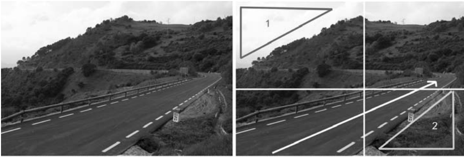
Photograph © Fernando Aida. GIASA digital archive. Regional Ministry of Public Works and Transport. Junta de Andalucía. Spain.
