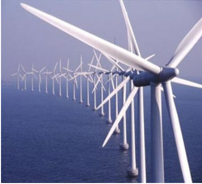
Fig. 1. An offshore wind farm
