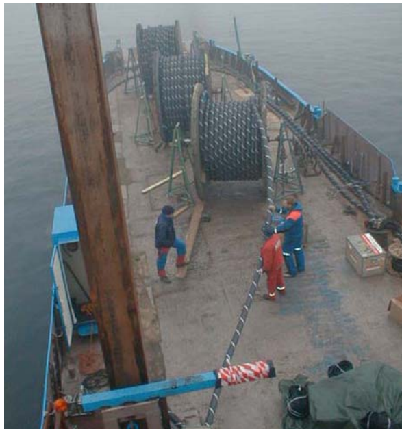
Fig. 7.7 Laying with cable drums on a barge
