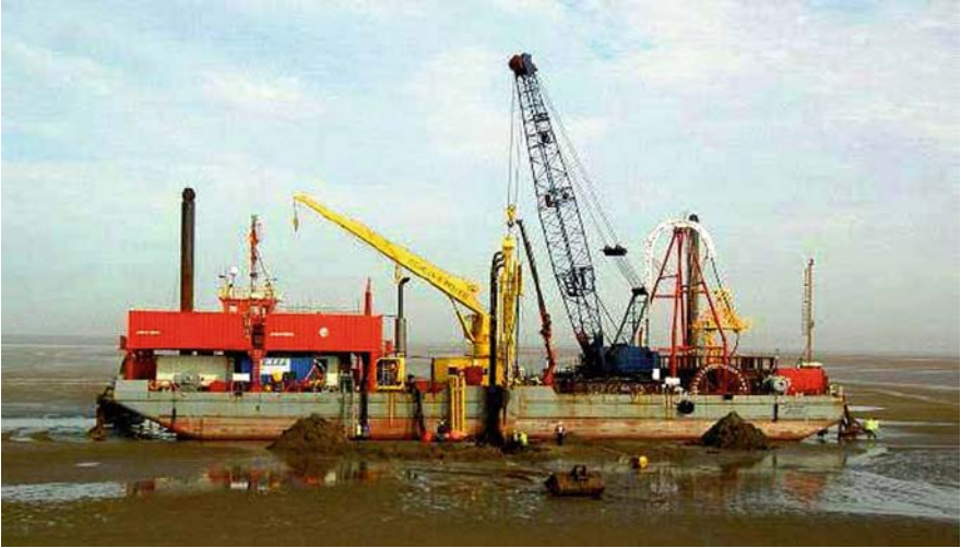
Fig. 7.3 Flat bottom barge mobilised for cable laying in tidal flats (Courtesy of Oceanteam Power and Umbilicals, UK)
