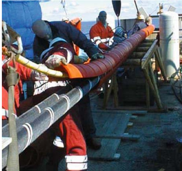
Fig. 7.23 Protective plastic shells are attached to two HVDC cables and an FO cable before the cable group leaves the vessel (Courtesy of ABB, Sweden)
