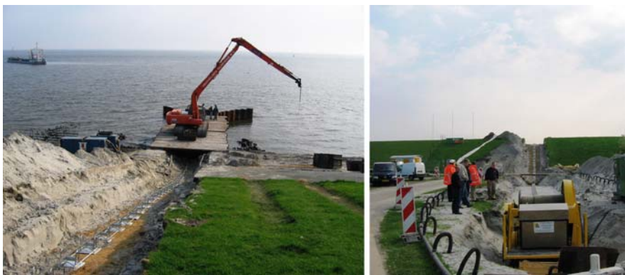
Fig. 7.14 Landing of a submarine power cable (NorNed) in open trench over the protection wall. In the splash zone, an open pit was created with cofferdam walls to receive the cable. The cut in the dike is visible in the distance in the right picture. Cable winch is in the foreground
