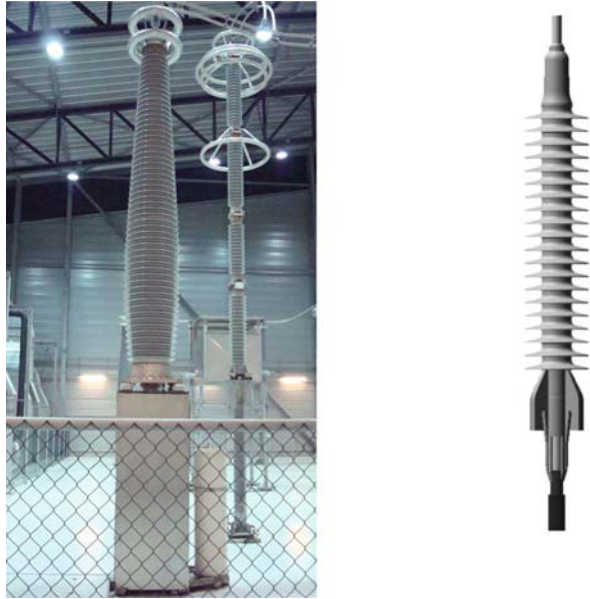
Fig. 4.8 Indoor HVDC cable terminations for mass-impregnated cable ( left ) and extruded cable ( right ). Small oil reservoir cylinder is attached to the stand of the left termination
