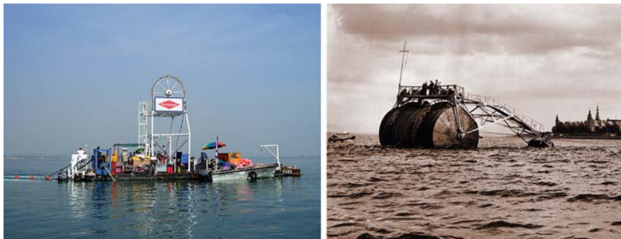
Fig. 11.3 (a) Purpose-built cable laying arrangement for calm waters. (b) Floating cable drum used as laying vessel. (Courtesy of NKT Cables A/S)
