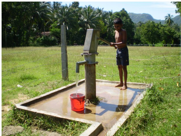
Fig. 7.15. There are millions of tube wells in Bangladesh, providing 95% of the drinking water in this country
