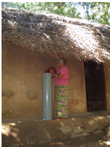
Fig. 4.21. Household defluoridator using burnt bricks distributed in villages in Sri Lanka
