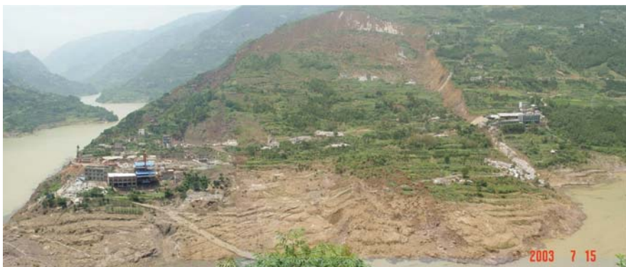
Fig. 8.3 Front-on view of the Qianjiangping landslide (taken by Y.M. Zhang, July 15, 2003)
