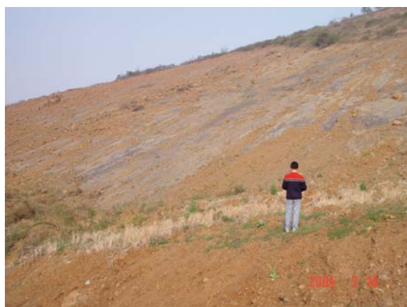
Fig. 8.5 The exposed planar sliding surface, which is also a sandstone bedding plane (there is a damaged rice paddy in front of the person)
