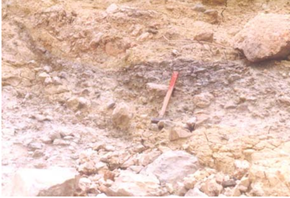
Fig. 3.18 Landslide zone in the front flank of the Huangtupo landslide, in the riverfront, 200 m to the west of Erdaogou
