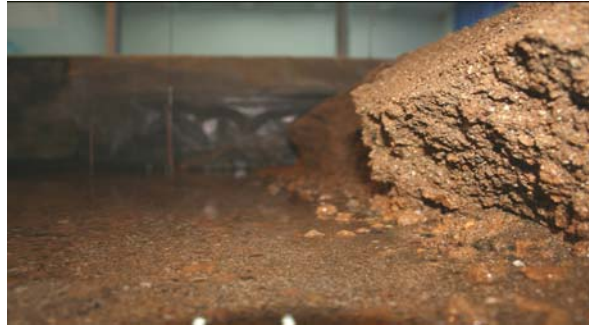
Fig. 27.16 The niche eroded by wave action on the back of the slope
