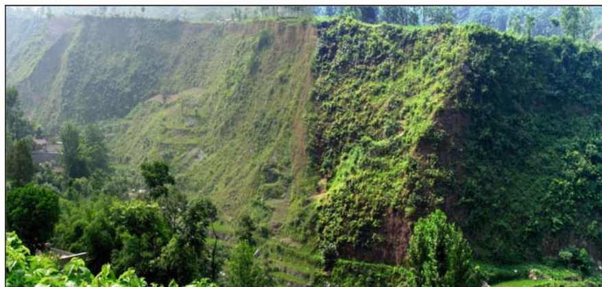
Fig. 13.9 High steep slope on the lower part of the left bank of the Bailuxi River
