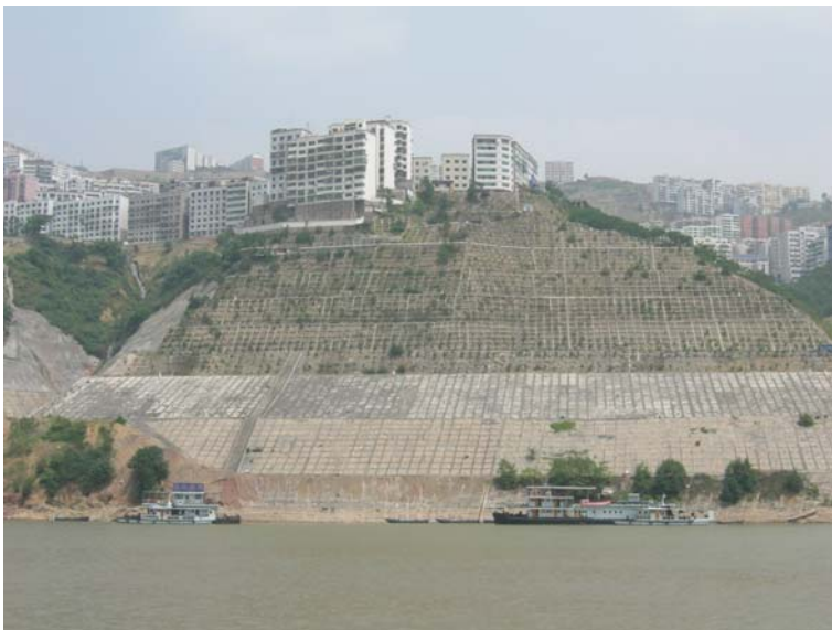
Fig. 24.6 Front view of the Yuhuange landslide in Wushan County
