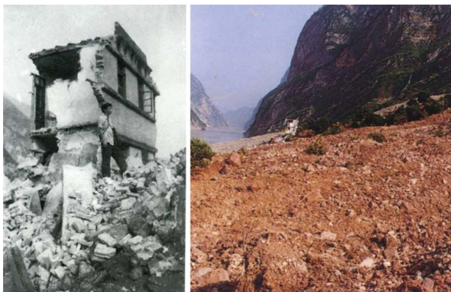
Fig. 18.4 Buildings destroyed by the landslide (Office building of the Rock Fall Survey Department of Xiling Gorge, Hubei Province)
