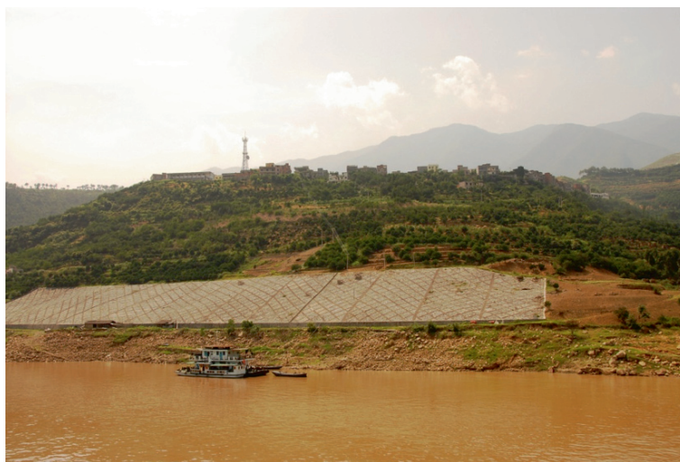
Photo 20 Countermeasure works applied to the landslide between Wu Gorge and Qutang Gorge
