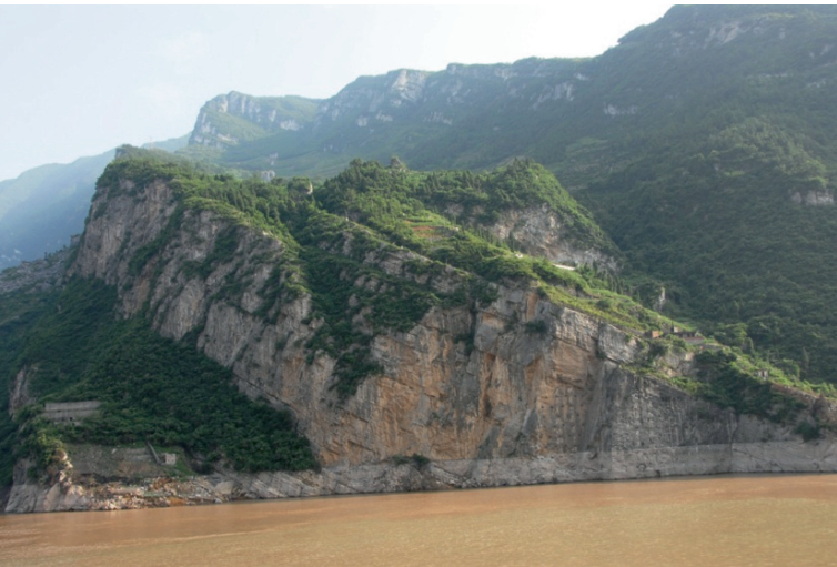
Photo 14 (Xiling Gorge western part) The Lianziya potential dangerous limestone cliff. It is located on the opposite bank of the Xintan landslide. Countermeasure works such as anchors were applied to reinforce the part near the river. This area is the narrowest part of the Three Gorges
