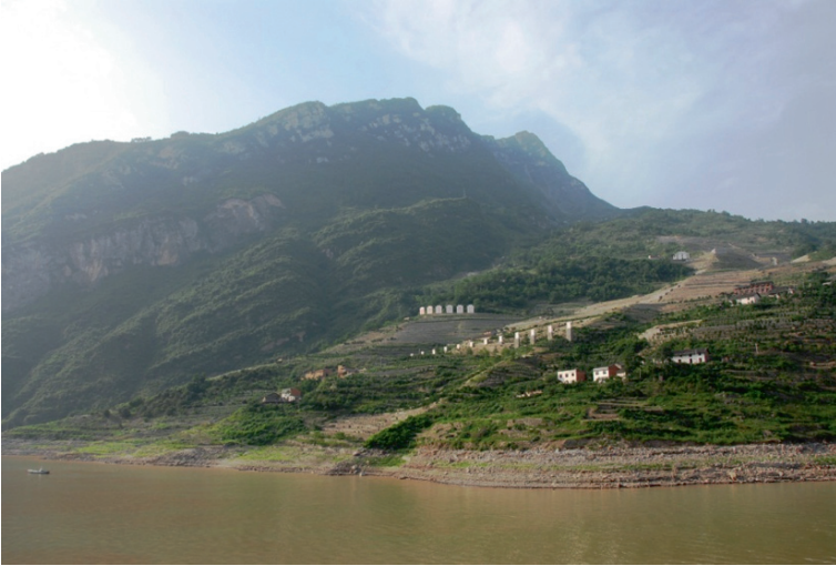
Photo 13 (Xiling Gorge western part) The site of the Xintan landslide that occurred in 1985. Because of the successful failure prediction based on monitoring, no one was killed by the large-scale landslide. It has been preserved as a visitor’s site for geo-hazard education, after the gradation was performed
