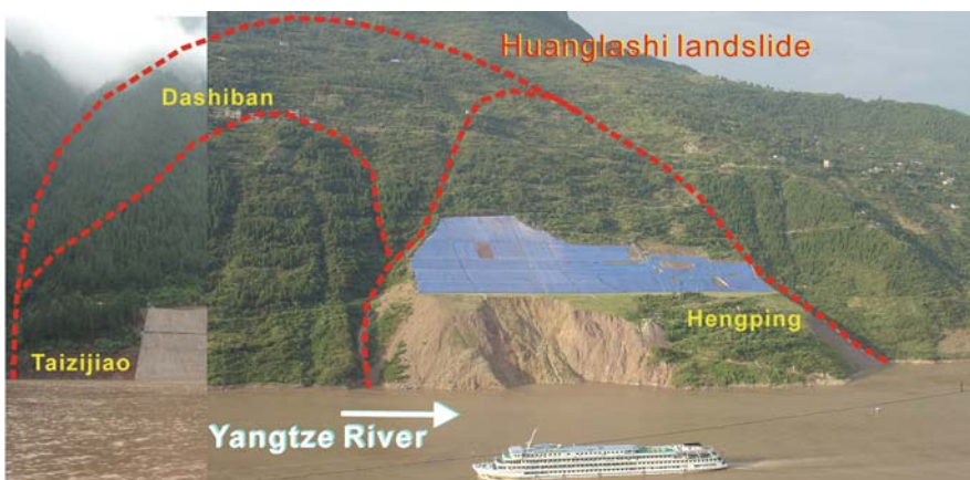
Fig. 22.1 Full view of the Huanglashi landslide
