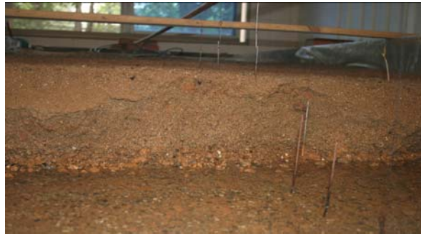
Fig. 27.17 The perpendicular wall after the collapse
