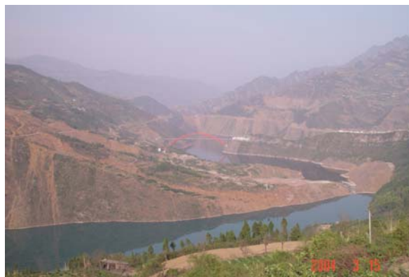
Fig. 8.2 View of the Qianjiangping landslide from the upstream side of Qinggan-he River (taken by F.W. Wang, March 15, 2004)
