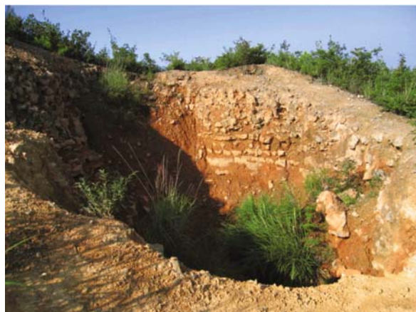
Fig. 4.9 Subsiding pit on the top of the dangerous rockmass
