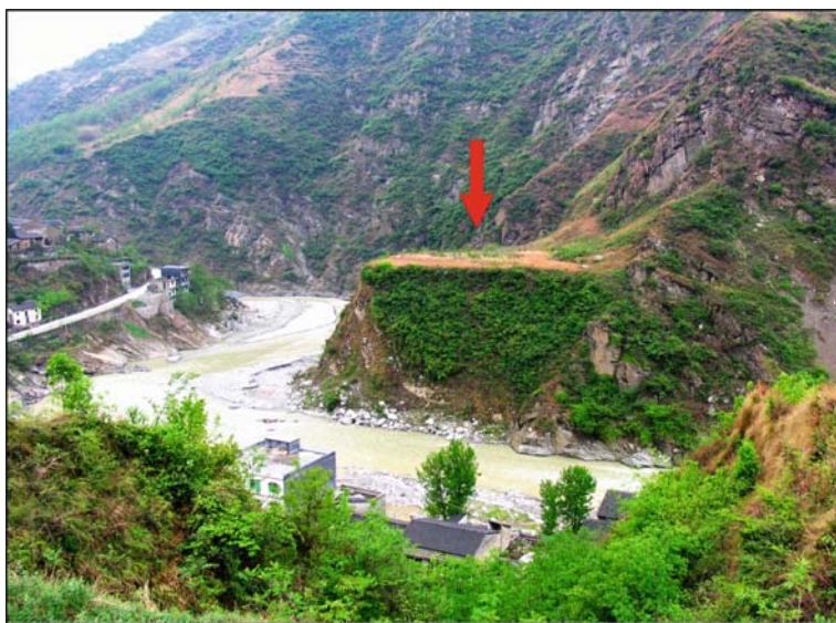
Fig. 13.3 Triangular-shaped dam residual once formed by the Bailuxi mud-rock flow stands on the right bank of the Daninghe River. Arrow indicates the top which is about 25 m above the water
