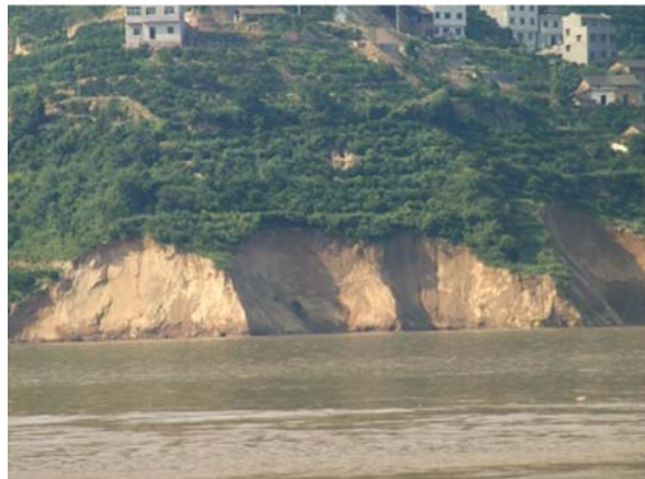
Fig. 5.2 Toe-erosion collapses (Huang et al. 2005)
