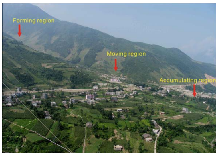
Fig. 13.4 View of Yangjiawan River mud-rock flow region
