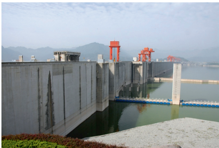
Photo 7 (Three Gorges dam) The Three Gorges dam
