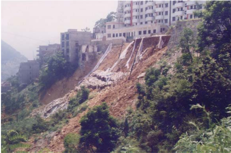
Fig. 15.14 Erdaogou landslide occurred on June 10, 1995. Note it developed in the debris accumulation. View is from the northwest
