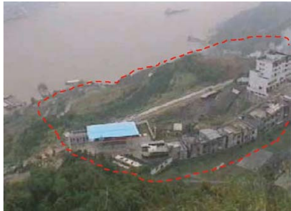
Fig. 20.2 Photograph of the Muzishu landslide (Dashed red line indicates landslide boundary)
