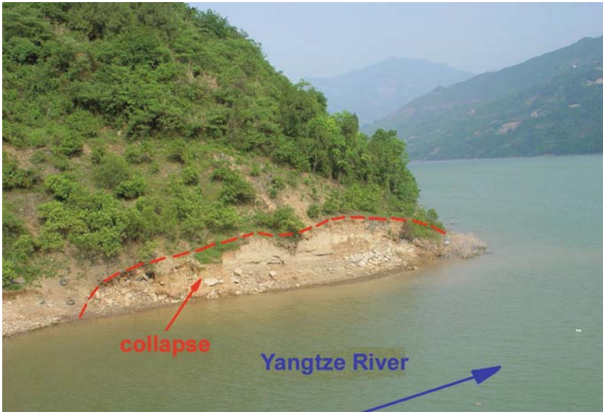
Fig. 16.12 Partial collapse of the landslide after the 135 m water level impoundment
