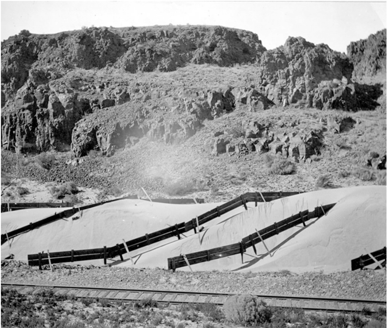
Fig. 23.2 Fences installed to guide drifting sand away from the railroad in the Columbia river gorge, near Grant, Oregon. Similar fences are sometimes found elsewhere to prevent blowing snow from blocking roads. USGS photo by G.K. Gilbert
