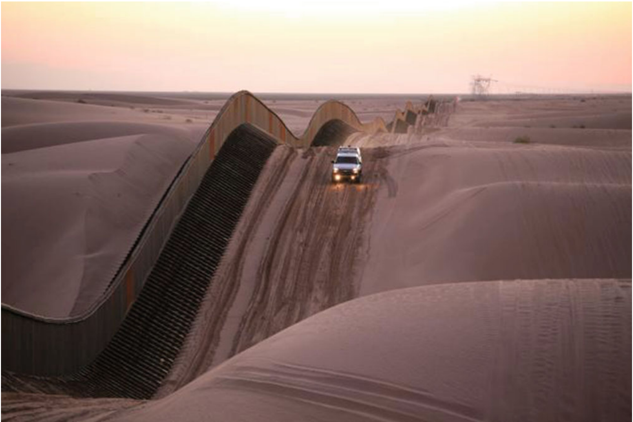
Fig. 23.9 The ‘floating fence’ at the US–Mexico border near Yuma, in the Algodones dunes. The fence is designed to maintain its height even as the sands shift beneath it. Photo by US Customs and Border Protection
