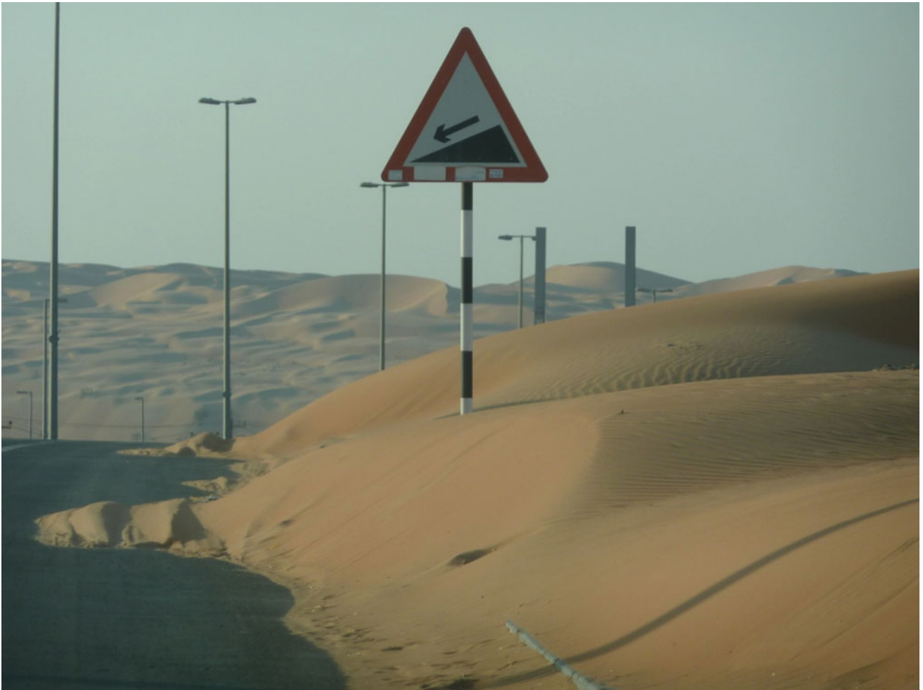
Fig. 23.7 Small barchanoid dunes intrude onto the road in the Liwa oasis, United Arab Emirates. This occurs preferentially on the top of megabarchan dunes, where the wind is accelerated and there are no date palms to trap the sand. Photo courtesy Jani Radebaugh
