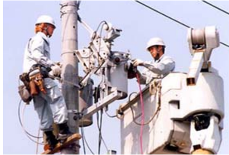
Fig. 1. Power distribution line maintenance Task performed by human workers
