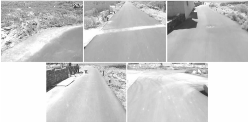
Fig. 1. Real aspect of the roads in the ITER facilities
