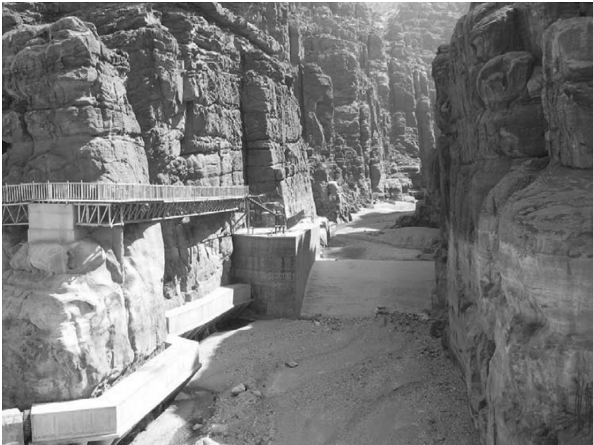
Fig. 2.1.8. Water capture with weir, intake building and deviation channel at the mouth of Wadi Mujib at the Jordan Dead Sea coast. The capture and deviation of surface water for domestic and agriculture water supply is one of the main reason for the current depletion of the Dead Sea water level (Foto: Hötzl).
