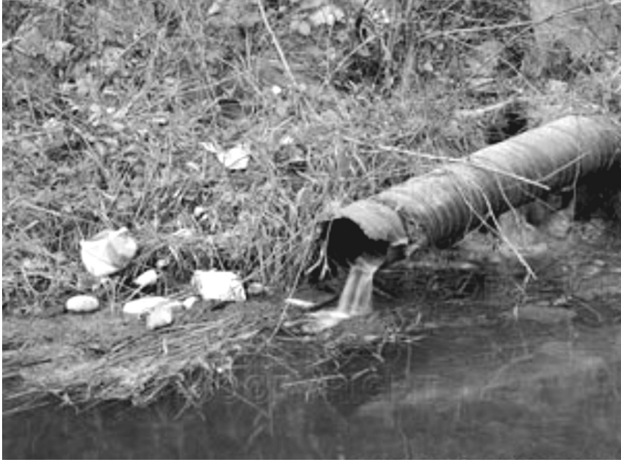
Fig. 3.10.2. Domestic wastewater draining into a creek.
