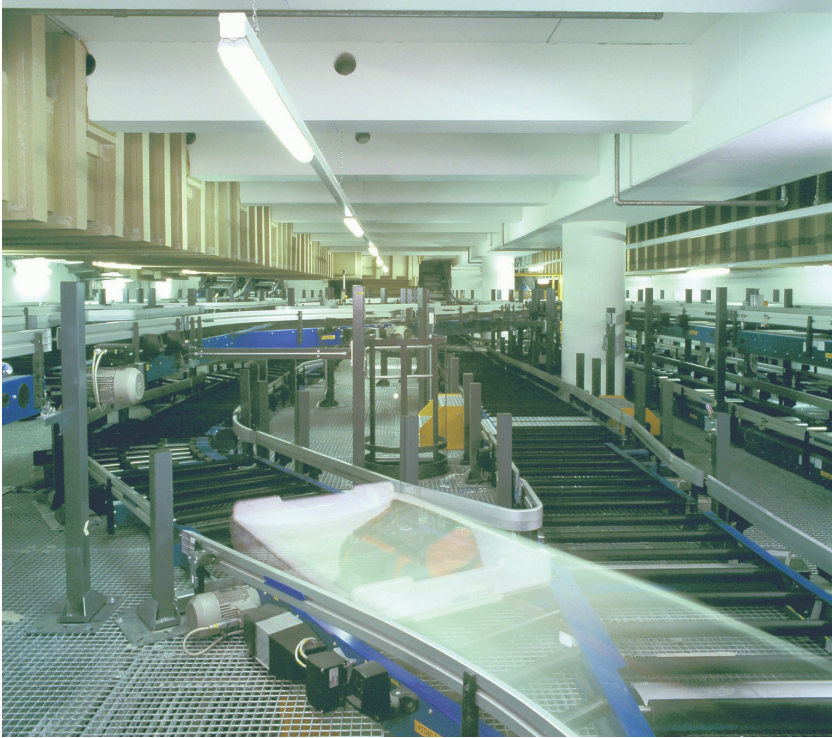
Fig. 1. Snapshot of a BHS with a moving tote containing a bag in the foreground
