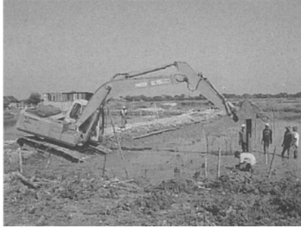
(a) Installation of bamboo piles
