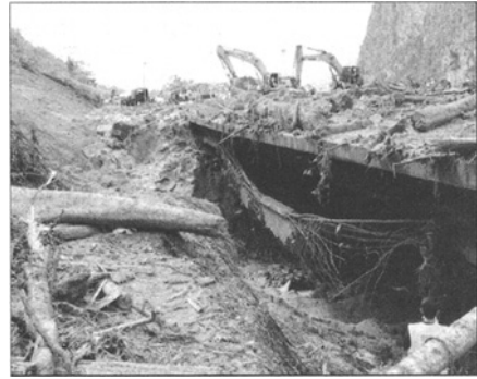
Figure 3. Accumulation of debris at bridge opening
