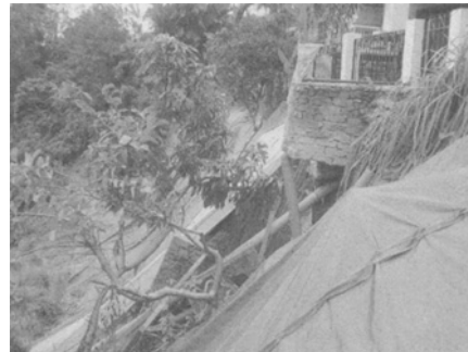
Figure 9. Drainage discharging into slope in 2004
