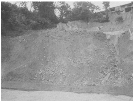
Figure 21. Laying of sand drainage layer
