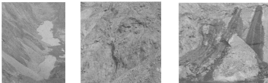
Figure 1. The exterior of slope footwall at Xinqiao mine
