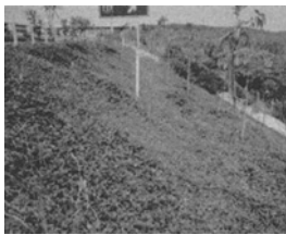
Picture 7. A stretch of trial embankment after construction
