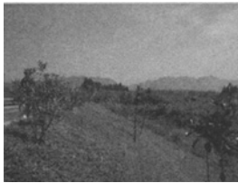
Picture 5. A stretch of trial embankment after construction
