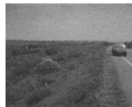
Picture 8. A stretch of trial embankment after construction
