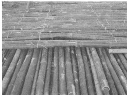
(b) Installation of bamboo mattress
