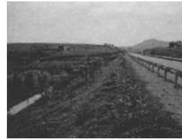
Picture 6. A stretch of trial embankment after construction
