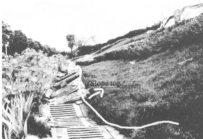
Figure 2. Lateral displacement and hunching
