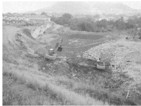
Figure 20. Rock-key of lower embankment
