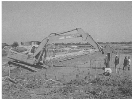
(a) Installation of bamboo piles
