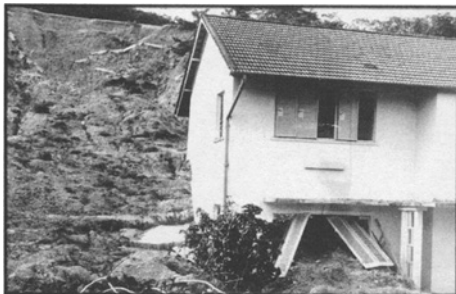
Figure 3. Landslide at quarters 1276
