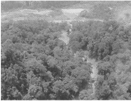
Figure 2. Aerial view of debris flow toward Bridge site
