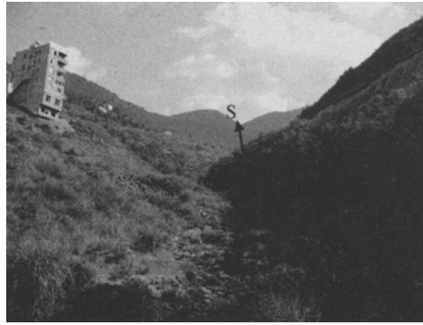
Figure 1. The picture of dumping site in Huangjia valley
