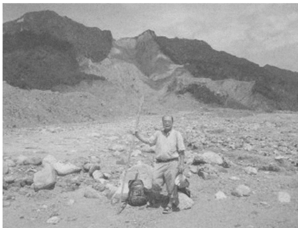
Figure 5. Colossal slope failure at Guinsaugon, Leyte
