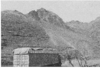
Figure 6. The slope in K2403+500 of G32020
