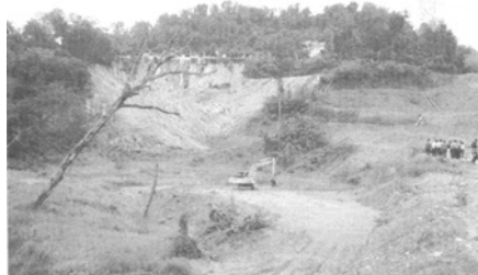
Figure 11. General view of landslide
