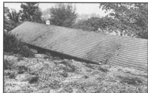
Figure 4. Landslide at quarters 1280
