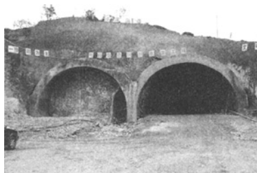
Figure 2. Yangwan tunnel in Jinliwen Expressway
