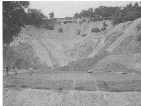
Figure 22. Construction of geogrid embankment
