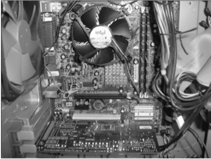
Fig. 7.3. View of the PC and the DS1104 board
