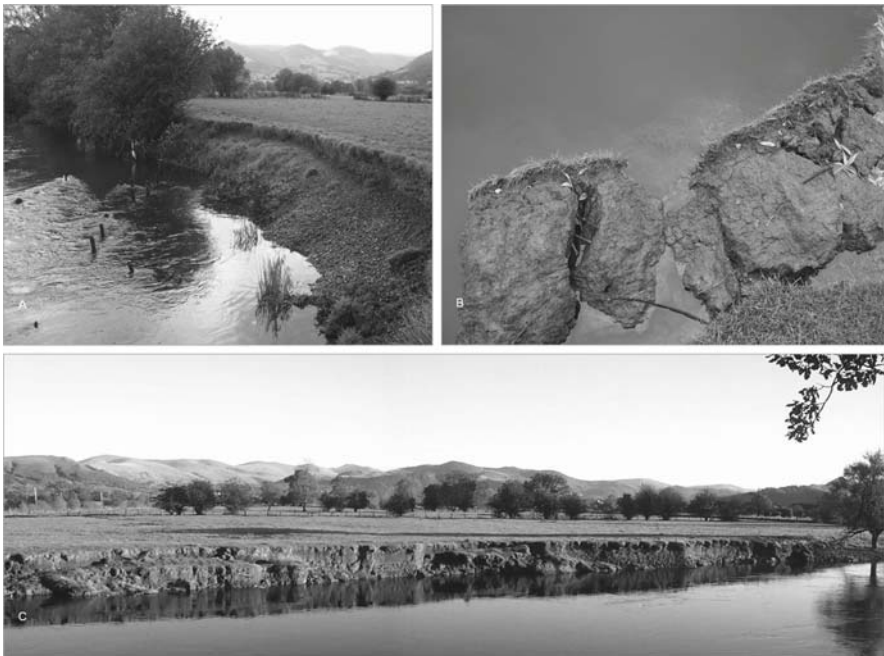
Fig. 6 Examples of bank failures on the lower Derwent. (a) Recent slumps involving fine upper bank sediments and gravel ( lower bank ). (b) Block failures of fine cohesive material. (c) Extensive bank erosion upstream of the Low Stocks Bridge monitoring site
