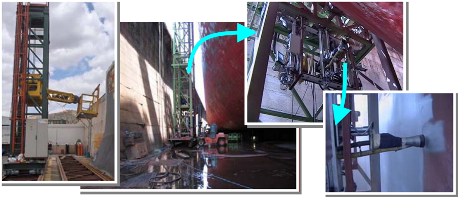
Fig. 2. XYZ table mounted on a crane. Tests in NAVANTIA shipyards.
