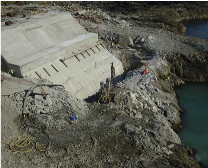
Fig. 7.41. Completion of the structural work
