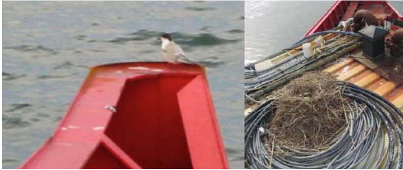
Fig. 7.86. Bird life in Nissum Bredning. An Arctic Tern perches on the tip of the reflector wing, and a Herring Gull has made its nest in some spare cable on the roof of the control room
