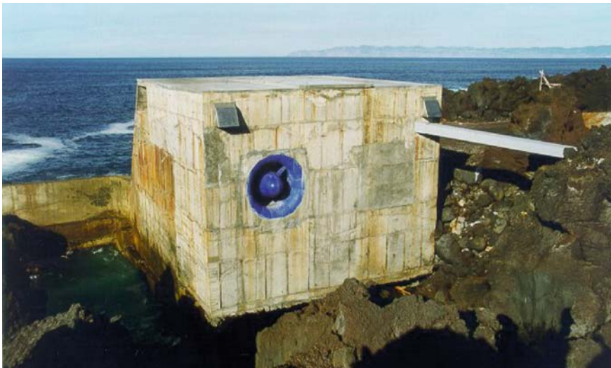
Fig. 7.8. Back view of the Pico Plant
