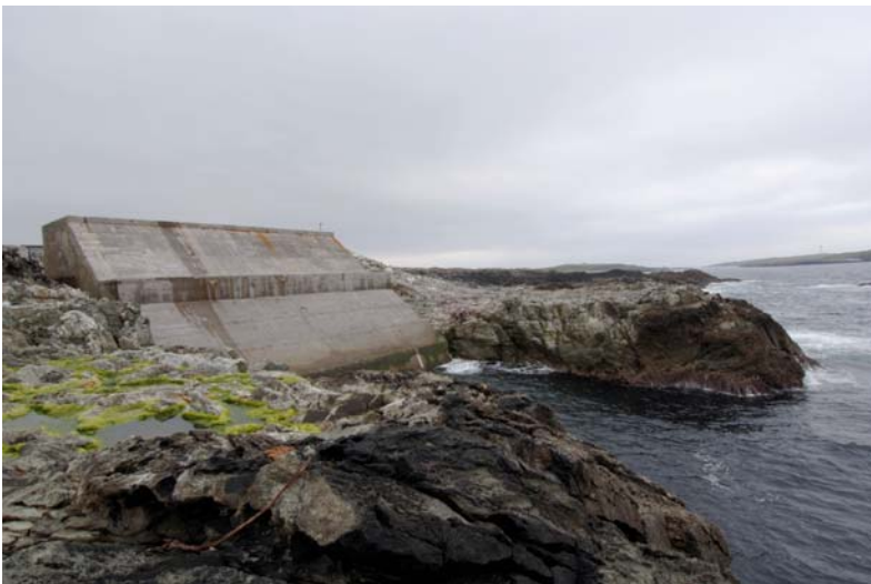
Fig. 7.38. LIMPET OWC operating on Islay since 2000
