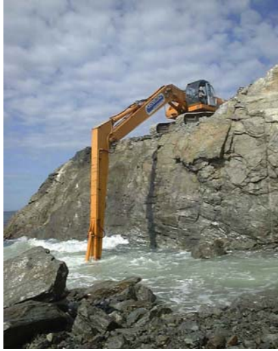
Fig. 7.42. Rock removal operations
