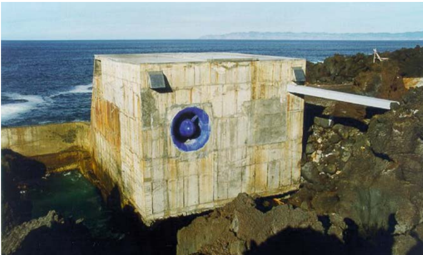
Fig. 7.8. Back view of the Pico Plant
