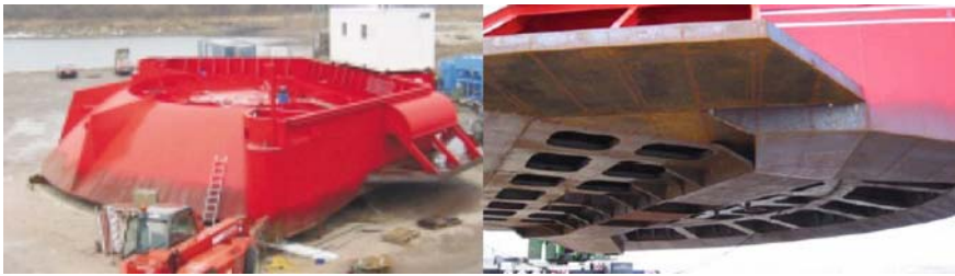
Fig. 7.72. The platform at the dockside in 2003 before being launched. On the right the open air compartments used for buoyancy regulation can be seen
