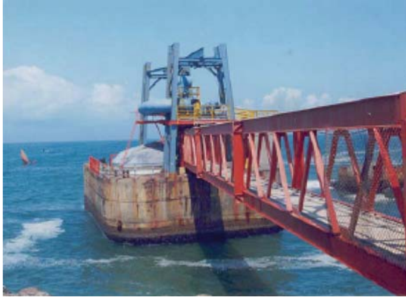
Fig. 6.62. Wave energy plant at Vizhinjam (Sharmila et al., 2004)
