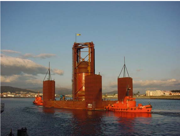
Fig. 7.55. View of AWS at the harbour of Viana do Castelo, Portugal
