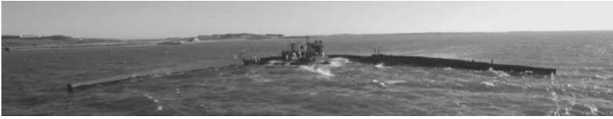
Fig. 7.25. The Wave Dragon prototype in Northern Denmark. The reservoir and ramp are situated in the middle, with the reflectors concentrating the waves towards the ramp
