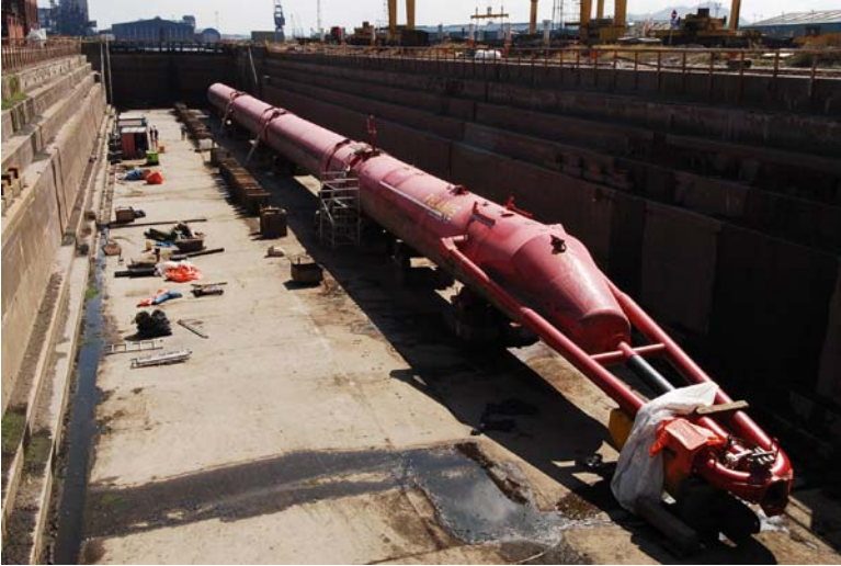
Fig. 7.66. The full-scale Pelamis prototype while being refitted in Leith (Edinburgh), 2006
