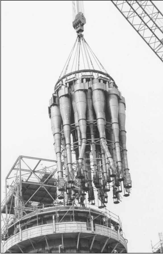
Fig. 16.2.9. A large 2-stage cyclone system typical of that used to collect catalyst entrained off of the fluidized bed of a fluid catalytic cracking unit (FCCU). Courtesy Emtrol LLC
