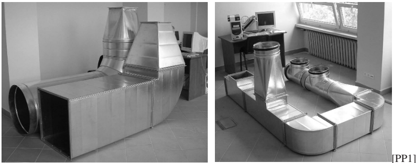
Fig.5. Ventilation ducts used as test stage
