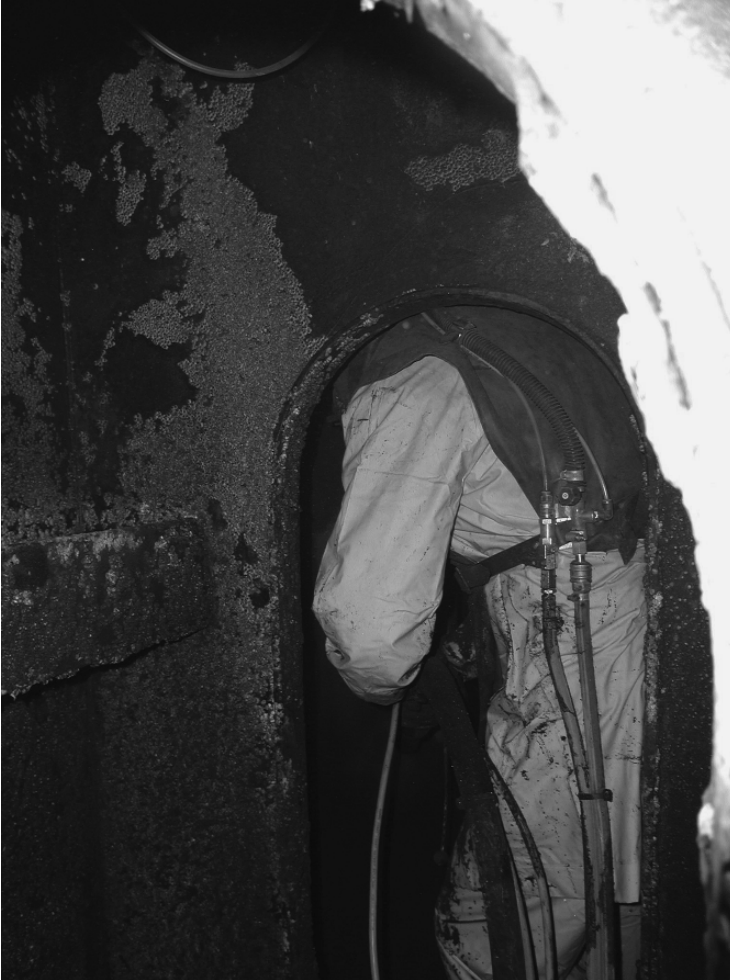
Fig. 7.24 Blast cleaning in a confined space (Photograph: Muehlhan AG, Hamburg)
