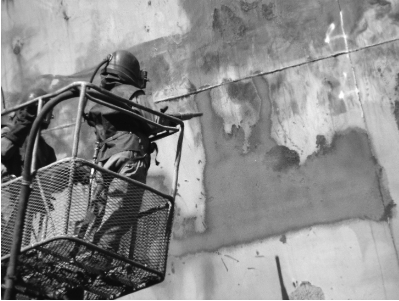
Fig. 7.22 Personnel protective equipment (Photograph: Muehlhan AG, Hamburg)
