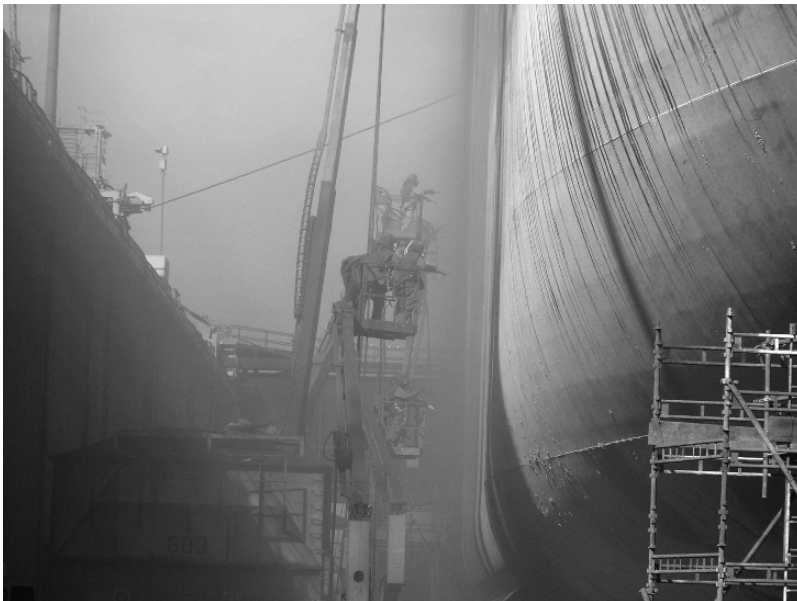
Fig. 7.7 Dust formation during dry blast cleaning (Photograph: Muehlhan AG, Hamburg)
