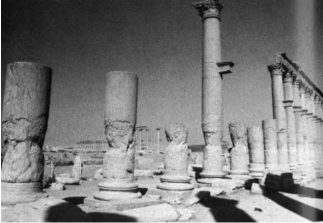
Fig. 1.1 The natural erosion (corrasion) of rock columns in Palmyra (Photograph: University of Tokyo)
