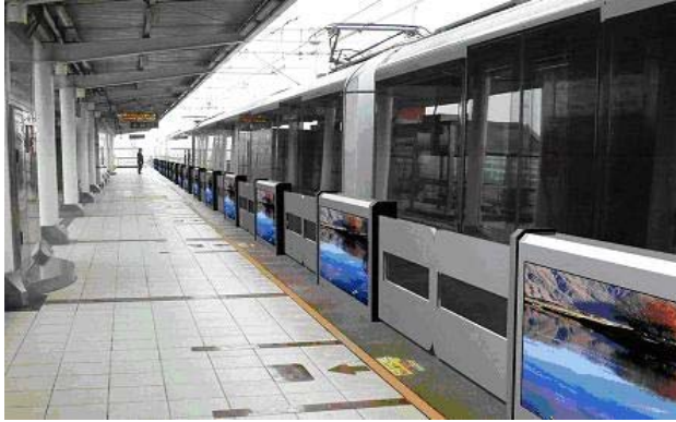
Fig. 1. Platform safety door of Chunshen Road Station, Light rail transit line No.5, Shanghai
