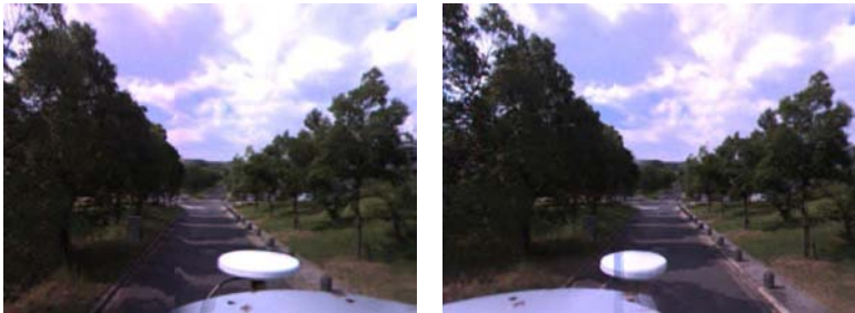
(iv)View of 180 degrees turned from going direction
