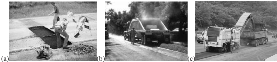
Fig. 3. M&R treatments: (a) Full-depth patching; (b) Hot recycling; (c) AC overlay
