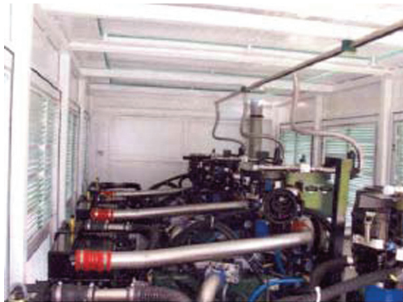
Fig. 7a.6 250 kW hydrogen genset
