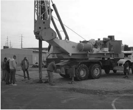
Fig. 12.14. A drilling rig drills the foundation hole
