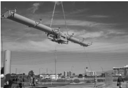
Fig. 12.16. Installation of the drive/torque tube assembly
