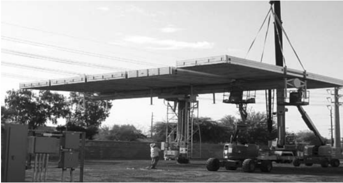
Fig. 12.18. The final module is installed on the torque tube
