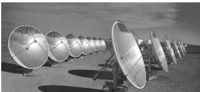
Fig. 1.14. Field of PV parabolic dishes manufactured by Solar Systems in White Cliffs, NSW (Australia). Each dish focuses the light on a compact actively cooled receiver, whose surface is a parquet of BPC cells. Each disk is rated 25 kW p nominal
