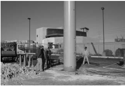
Fig. 12.14. A drilling rig drills the foundation hole
