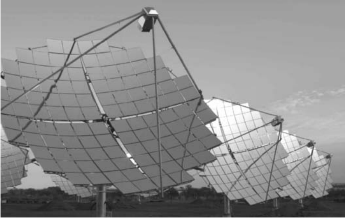
Fig. 3.2. Hermannsburg, Australia, 190 kW power station, with SunPower back contact solar cells in the receiver at the focus. (Courtesy Solar Systems)
