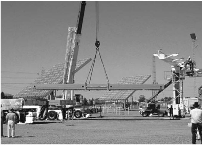
Fig. 12.17. A crane lifts the first module from the truck to the torque tube
