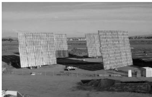
Fig. 1.13. Two-axes tracking arrays from AMONIX, installed at Arizona Public Service, Scottsdale. They use 27% efficient BPC solar cells operating at 250 \times under point focusing laminated Fresnel lenses: the nominal array power is 25 kW. This technology was licensed to GUASCOR-FOTON (Spain) in 2005 and is currently being commercialized
