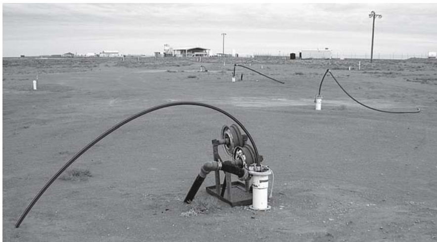
Fig. 6.4. Borefield of the Honeymoon ISL uranium mine, Australia. An acid leaching process is applied to a confined aquifer
