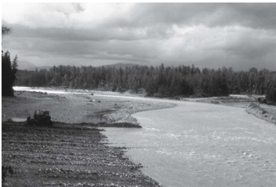
Fig. 4.8. Earthworks in the Ajkwa River, Irian Jaya, Indonesia. Tailings are discharged (~8.7 Mt per year) from the giant Grasberg-Ertsberg mine into the Ajkwa River, causing severe aggradation and flooding of vegetated lowland downstream of the mine. Areas inundated with tailings are to be turned into productive and sustainable agricultural land
