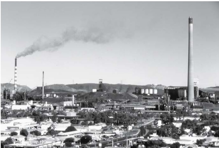
Fig. 1.10. The copper and lead smelter stacks at Mt. Isa, Australia. Until recently, the sulfurous plume was dispersed over the town and across 100 000 km 2 northwest of Mt. Isa. Over the years, the emissions resulted in the acidification of local soils and killed or reduced vegetation in the vicinity of the smelters. The recent installation of a sulfuric acid plant has reduced sulfur emissions
