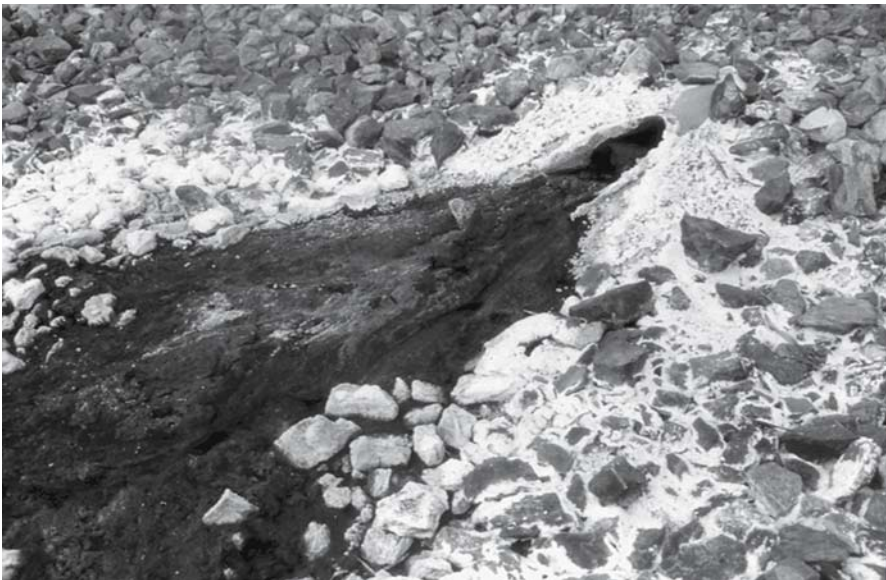
Fig. 2.17. Scalded seepage area at the base of White's waste heap (Fig. 2.16). The clay seal has cracked, and water infiltration into the dump has increased since the installation of the cover in 1984. Saline, acid seepages emanate from the base of the dump and precipitate abundant sulfate and iron oxyhydroxide efflorescences
