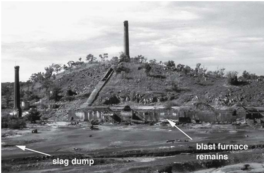
Fig. 1.4. Derelict copper-lead-gold-silver smelting works at Chillagoe, Australia. Smelting operations were conducted from 1901 to 1943 and produced 1 Mt of slag. The slag contains wt.% levels of zinc that is principally hosted by glass, olivine and hedenbergite
