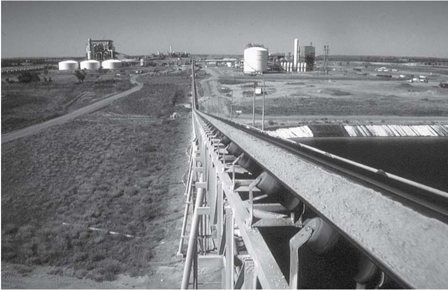
Fig. 7.4. View of parts of the fertilizer production facility at Phosphate Hill, Australia. Ammonia plant ( far right ), phosphoric acid facility ( centre ), granulation plant ( left ), and rail loadout facility ( far left ). A conveyor belt delivers phosphogypsum to the stack
