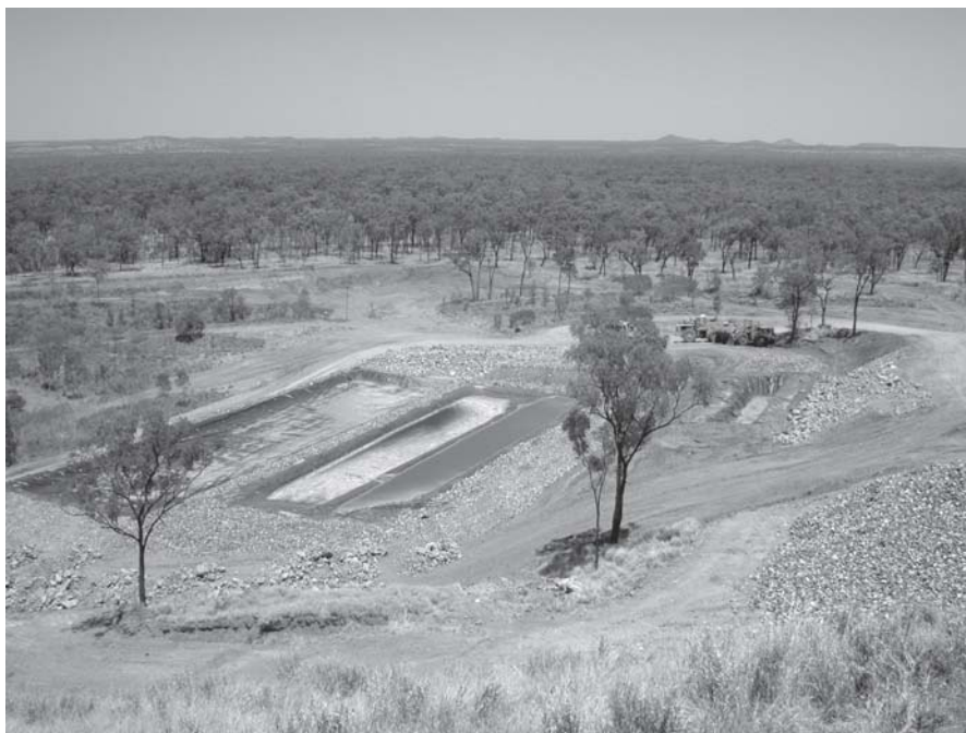
Fig. 5.5. Collection of cyanide-bearing seepage waters in shallow ponds at the base of the tailings dam, Red Dome gold mine, Australia. UV radiation causes the destruction of dissolved Cu cyanide complexes, precipitation of cyanate salts and attenuation of total cyanide from 300 \text{ mg l}^{-1} to <1 \text{ mg l}^{-1} in the successive ponds
