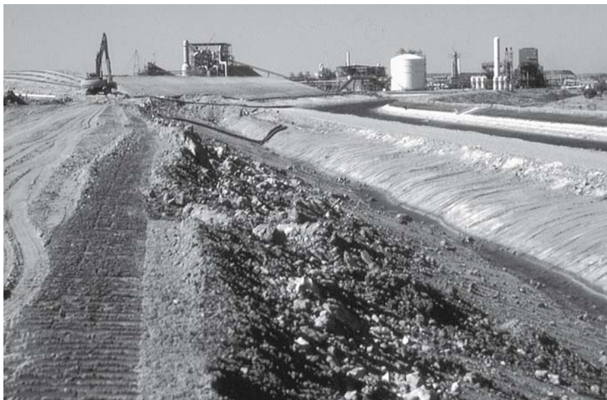
Fig. 7.5. Phosphogypsum stack at the Phosphate Hill mine, Australia. The dry phosphogypsum is reslurried prior to disposal and discharged onto the top of the stack where the solids settle. Waters (pH 1.5) seep through the stack and are collected in circumscribing plastic lined ditches
