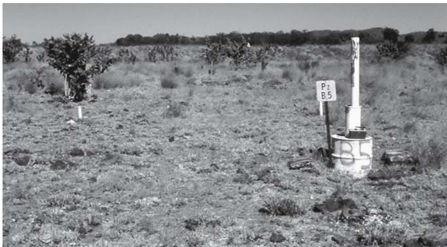
Fig. 6.7. Rehabilitated tailings dam at the Mary Kathleen uranium mine, Australia. The tailings dam has been rehabilitated using a multi-barrier system (clay and waste rock layers, vegetation cover). Piezometers allow sampling and monitoring of tailings liquids
