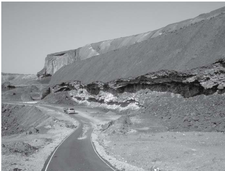
Fig. 2.8. Face of the Río Tinto smelting slag dump, Spain. Mineral efflorescences commonly occur as white sulfate salt precipitates (gypsum, epsomite, hexahydrate, bloedite, copiapite, roemerite) in protected overhangs and at seepage points at the base of the slag dump. The slags generate ephemeral drainage, which runs from the dump into the Río Tinto and contributes to its acidification and metal load
