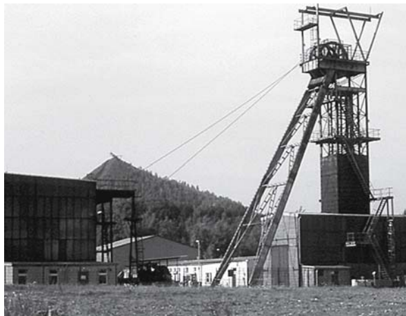
Fig. 6.2. Headframe of the Ronneburg underground uranium mine, Germany. Waste rock pile of uraniferous, carbonaceous shale is present behind the headframe
