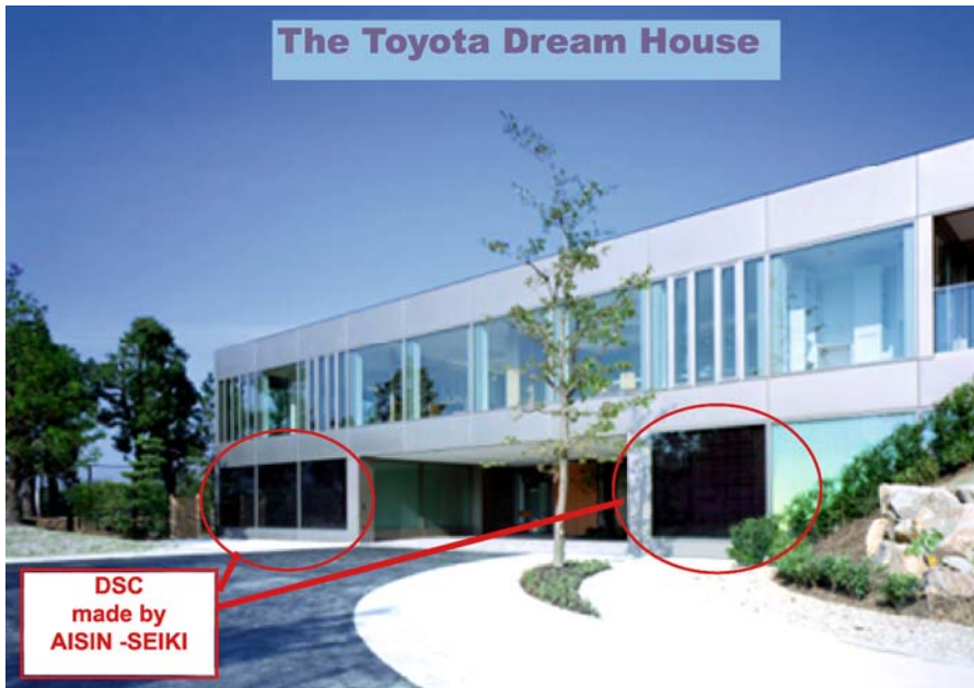
Fig. 23 The Toyota “Dream House” featuring DSC panels made by Aisin Seiki
