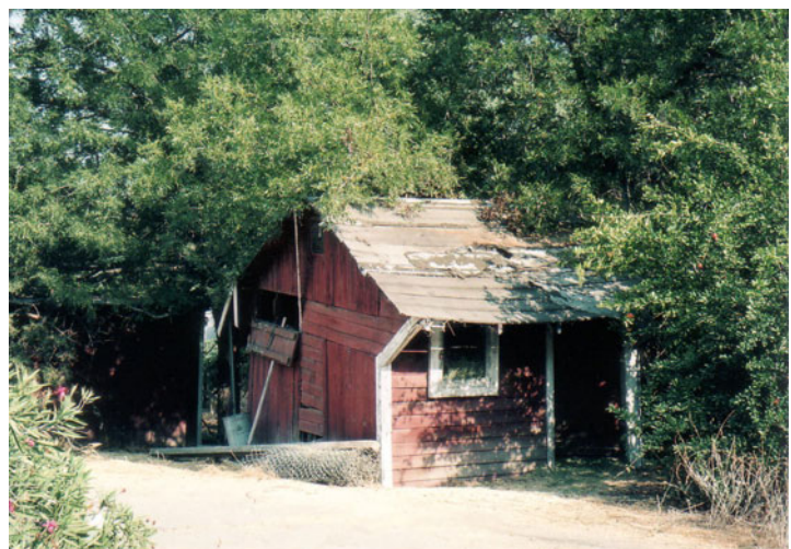
Fig. 7.4 A small hut that survived the 1994 Northridge earthquake
