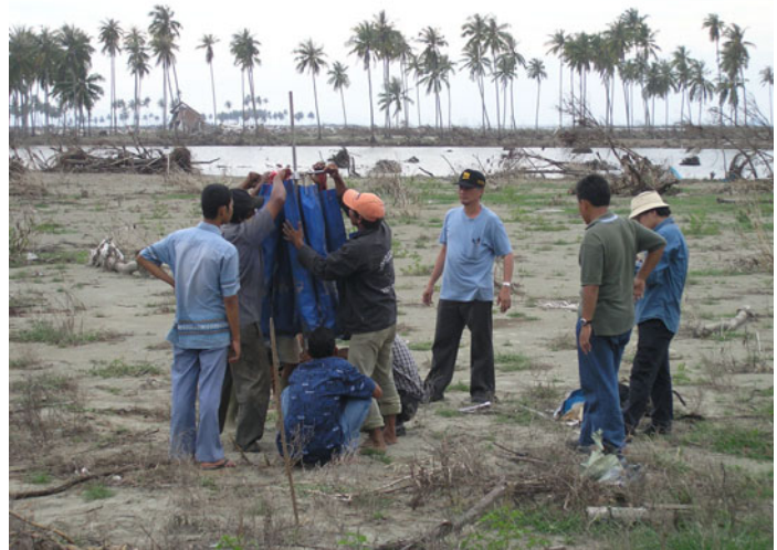
Fig. 5.45 Subsurface investigation by Swedish weight sounding supervised by Dr. Ilyas Suratman of Bandung Institute of Technology (Banda Aceh in Sumatra, Indonesia)
