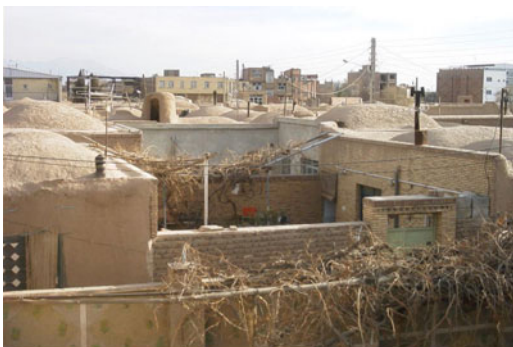
Fig. 5.38 Heavy roof of traditional house in Kerman, Iran
