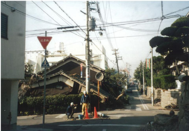
Fig. 5.28 Damaged shape of Japanese traditional house in Kobe
