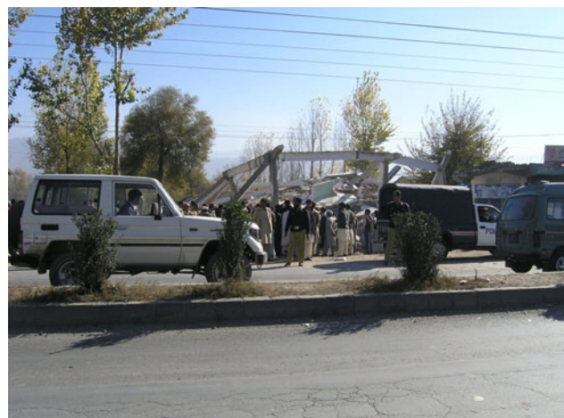
Fig. 5.44 Ruin of building which collapsed suddenly upon minor aftershock
