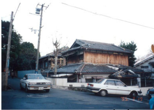
Fig. 5.30 Undamaged wooden house in Kobe (1995)
