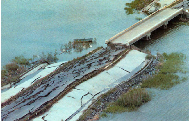
Fig. 14.11 Slump failure of road embankment due to subsoil liquefaction (Akita Sakigake Newspaper)
