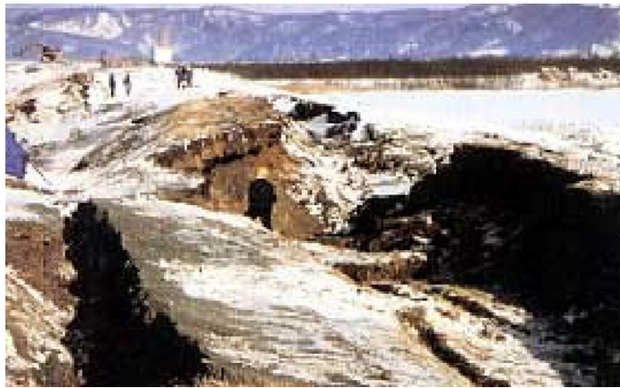
Fig. 14.11 Slump failure of road embankment due to subsoil liquefaction (Akita Sakigake Newspaper)
