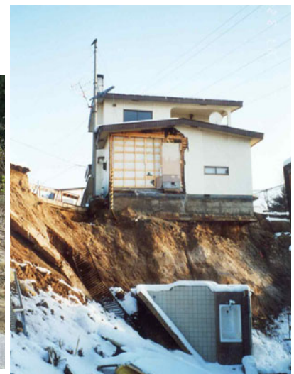
Fig. 14.10 Slip failure of fill part in cut-and-fill area (Midoriga-oka in Kushiro)
