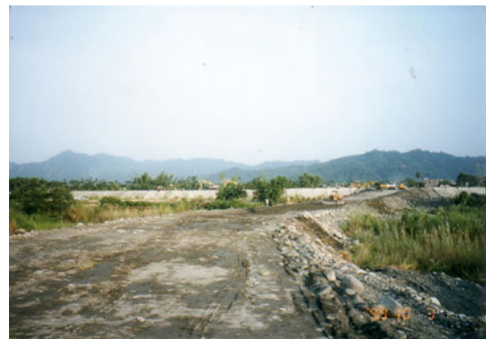
Fig. 14.22 Quick construction of temporary road embankment after collapse of bridge (1999, Taiwan)
