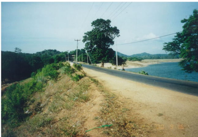
Fig. 14.41 Good condition of ancient irrigation dam in Sri Lanka
