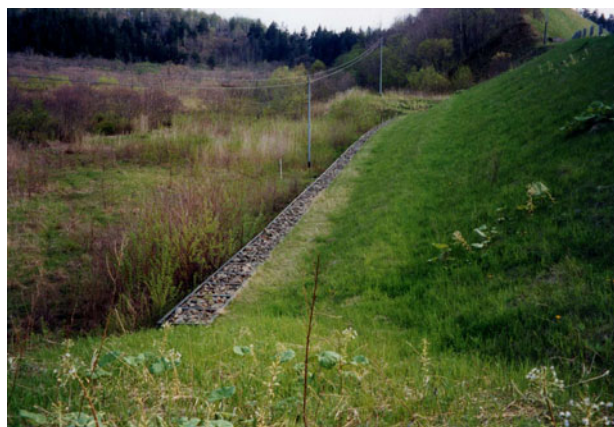
Fig. 14.46 Repaired toe of road embankment in Itoizawa (photo by T. Honda)
