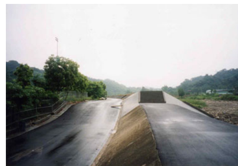
Fig. 14.3 Repaired shape of dike in Wufeng
