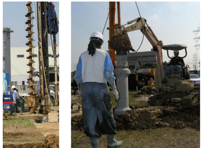
Fig. 13.32 Installation of nodular pile
