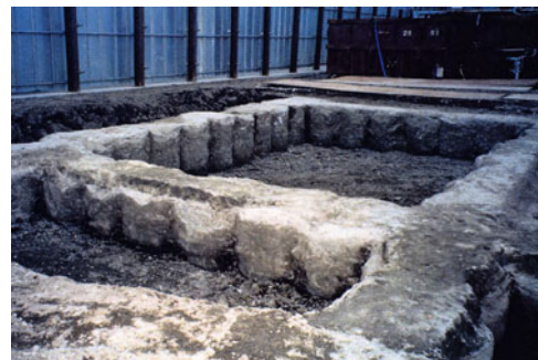
Fig. 26.111 Appearance of lattice structure immediately after installation (photograph by Takenaka Corporation)
