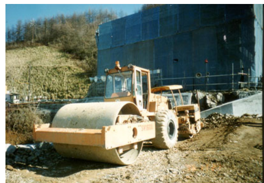
Fig. 17.29 Soil compaction for dam construction
