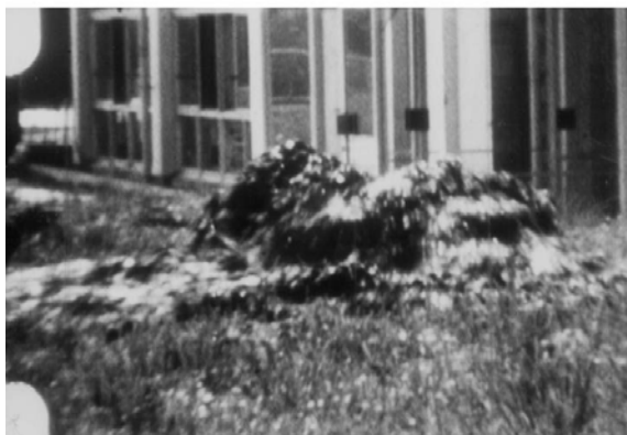
Fig. 25.59 Subsidence of Niigata Airport terminal building into liquefied subsoil (from motion picture by Mr. F. Yuminamochi)
