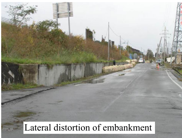
Fig. 14.4 Effects of collapse of road embankment on embedded lifelines
