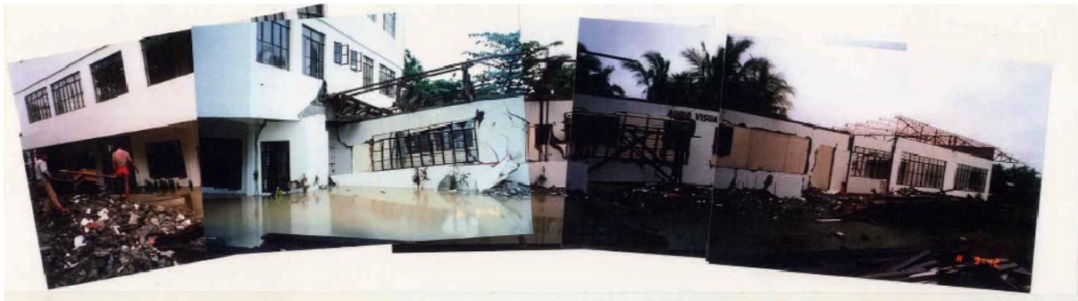
Fig. 17.4 Reduced subsidence of lighter annex
