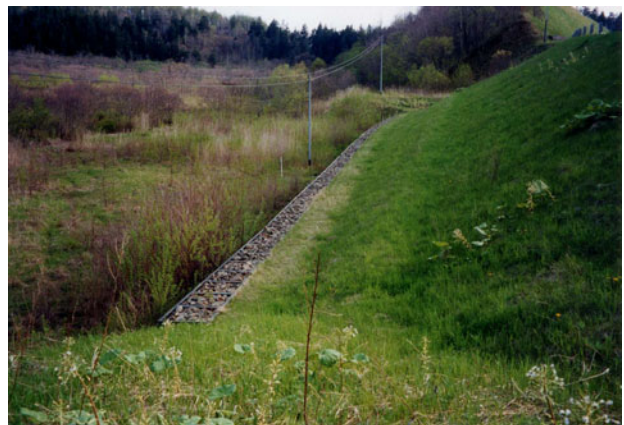
Fig. 14.46 Repaired toe of road embankment in Itoizawa (photo by T. Honda)
