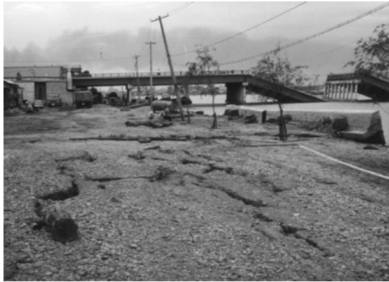
Fig. 17.20 Sheet pile wall near Showa Bridge in Niigata, 1964 (Dept. Civil Engineering, University of Tokyo)
