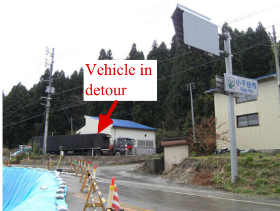
Fig. 14.25 Quick construction of temporary road next to the site of Fig.14.24
