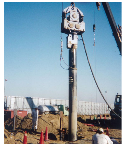
Fig. 18.15 Field shaking test for verification of drain pipe technology
