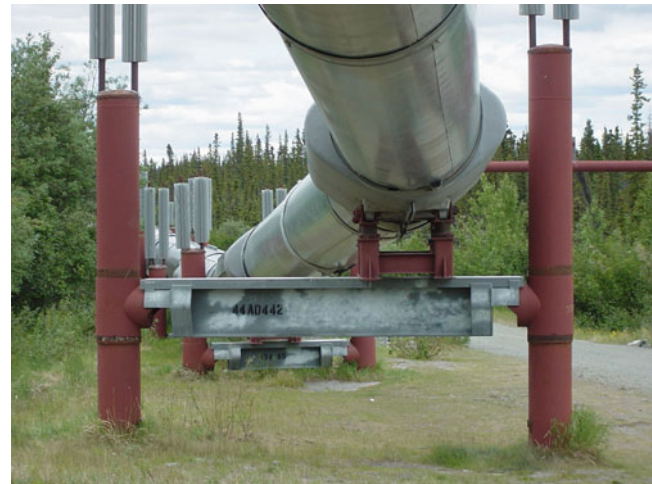
Fig. 16.25 Alaska pipeline which is simply sitting on lateral bar without fixing (Photo by M. Yoshimine)
