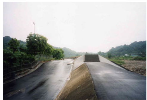
Fig. 14.3 Repaired shape of dike in Wufeng
