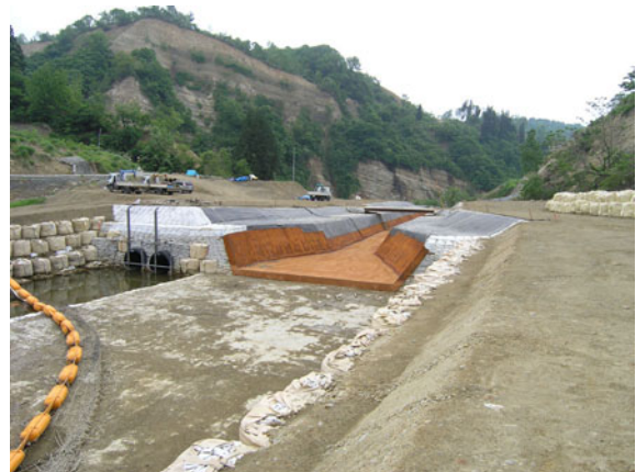
Fig. 15.29 Water drainage channel in Terano natural dam in Niigata
