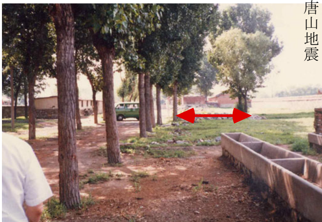
Fig. 16.16 Lateral displacement difference caused by Tangshan earthquake in China (Photo by Building Research Institute of China)
