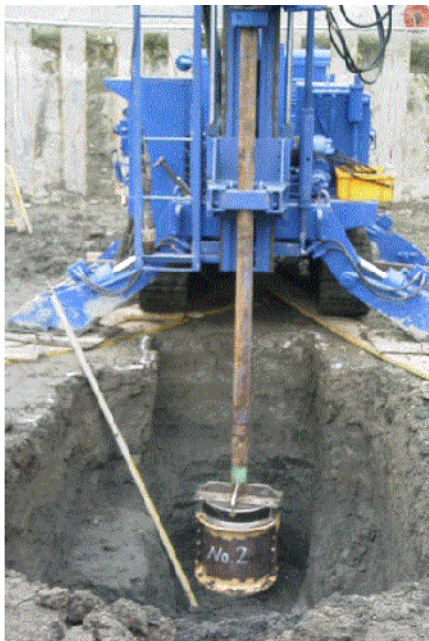
Fig. 10.60 Large block sampling of Yurakucho sand in Tokyo by Fujiwara et al. (2005)
