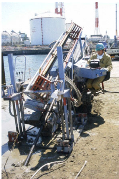
Fig. 26.119 Inclined drilling of bore hole for grouting under existing structure (Toa Corporation)
