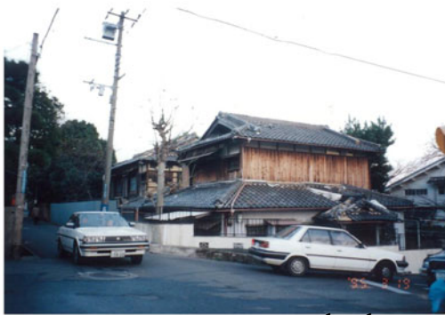
Fig. 5.30 Undamaged wooden house in Kobe (1995)
