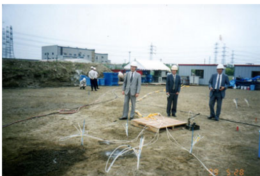
Fig. 26.116 Injection of silica liquid through multiple tubes into sandy ground
