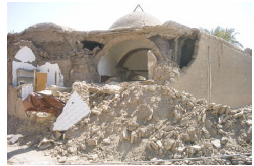
Fig. 7.14 Collapse of adobe house in Bam, Iran, in 2003
