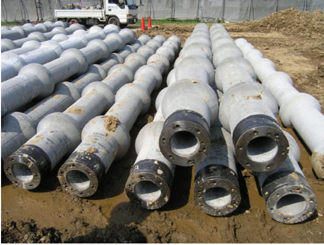
Fig. 13.31 Nodular piles prior to installation
