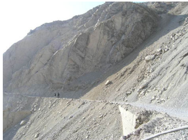
Fig. 15.6 Surface failure of weathered limestone slope near Muzaffarabad, Pakistan, in 2005
