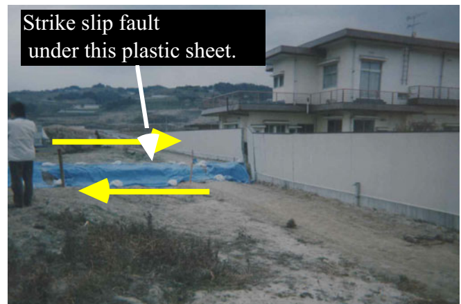
Fig. 16.17 Strike-slip fault passing under house (in Awaji Island, 1995)
