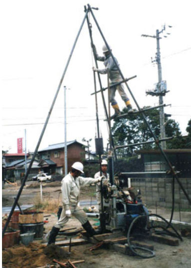
Fig. 8.10 Practice of standard penetration test
