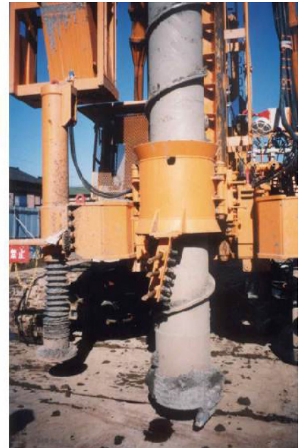
Fig. 26.86 Construction machine for gravel drain
