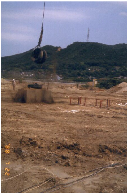
Fig. 26.67 Impact on ground surface made by free fall of weight (at Mizushima)
