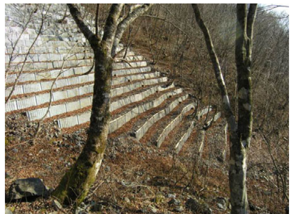
Fig. 15.13 Tree planting in unstable Ohya slope
