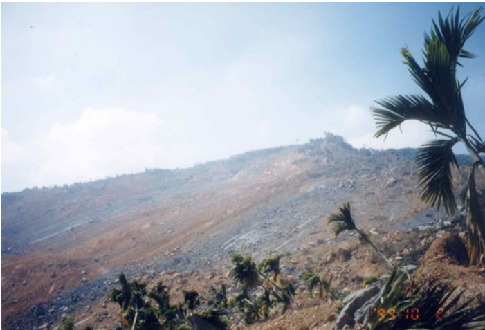
Fig. 15.37 View of Jiu-Feng-Er-Shan landslide
