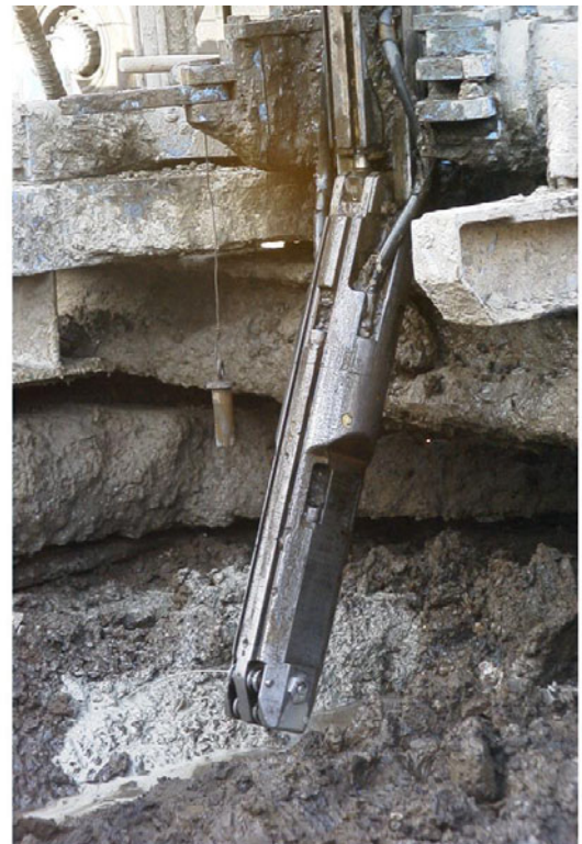
Fig. 27.8 Soil improvement of peaty material by grouting special liquid
