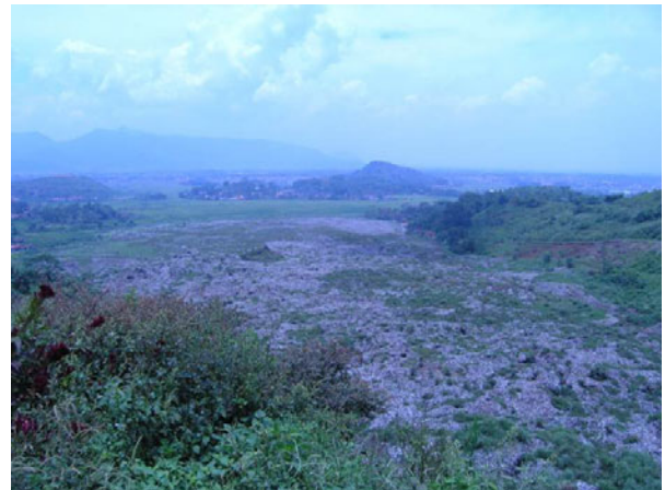
Fig. 10.74 Failure of Leuwigajah landfill near Bandung, Indonesia
