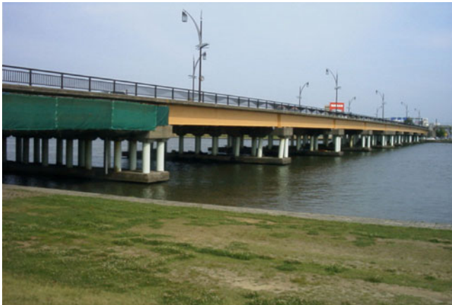
Fig. 24.65 Present foundation of Showa Bridge after reconstruction
