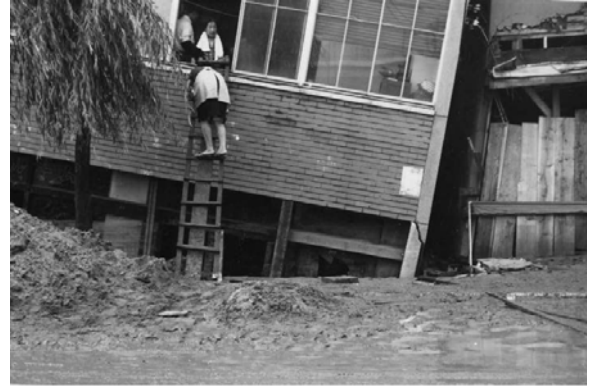
Fig. 17.51 Tilting of building in liquefied area in Niigata, 1964 (Department of Civil Engineering, University of Tokyo)
