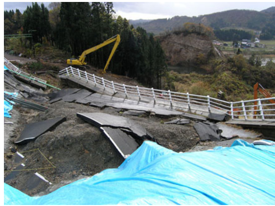
Fig. 14.24 Significant subsidence of road embankment resting on small valley topography caused by 2004 Niigata-Chuetsu earthquake
