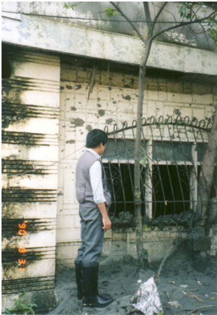
Fig. 18.4 Ejected sand on wall (Dagupan, 1990)
