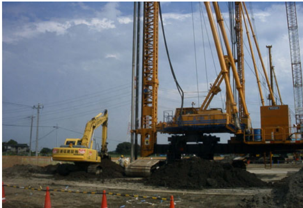
Fig. 26.104 Construction machine for deep mixing method
