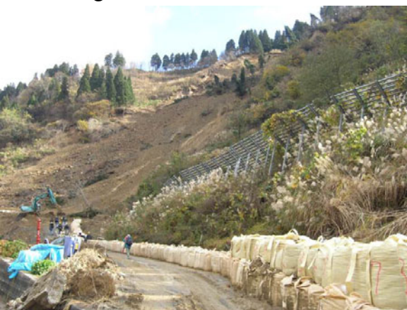
Fig. 13.26 Landslide near the western entrance of Haguro Tunnel
