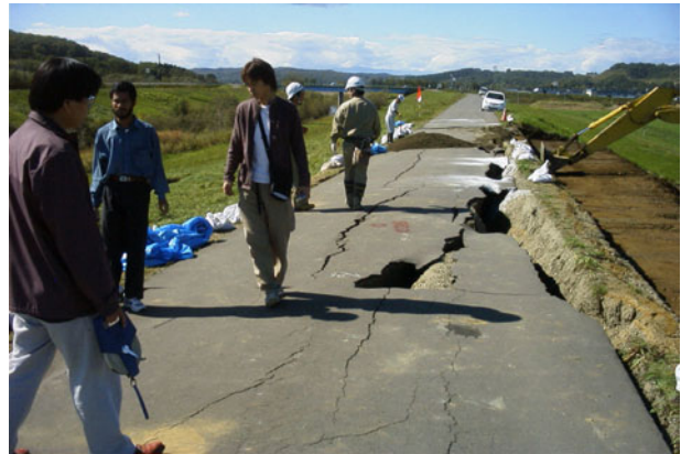
Fig. 17.14 Quick restoration after 2003 Tokachi earthquake
