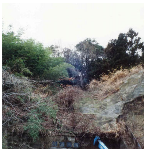
Fig. 13.22 Mountain behind entrance of Kinoura tunnel
