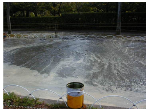
Fig. 17.41 On-going liquefaction and sand boiling in Yonago City (Photo by Mr. Naoki Higuchi)
