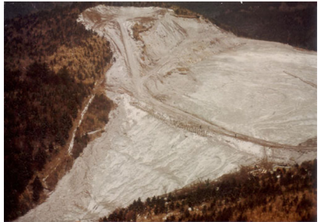
Fig. 20.20 Seismic failure of Mochikoshi tailing dam (Geotech. Engrg Lab., Univ. Tokyo)
