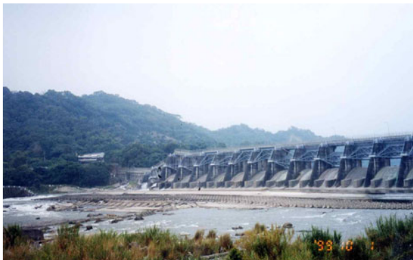
Fig. 16.9 Destroyed Shih-kang Dam
