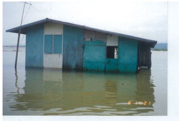
Fig. 16.58 Subsidence of Narbakan Peninsula due probably to densification of loose and young sandy deposit
