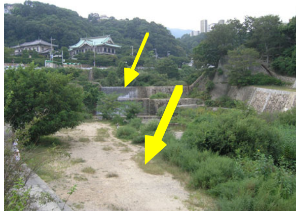
Fig. 26.5 Dams of debris in river channel
