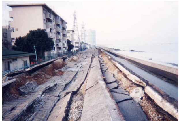
Fig. 17.35 Collapse of Yodo River dike in 1995 (Fudo Tetra Corp.)
