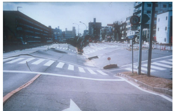
Fig. 13.5 Ground subsidence above Daikai subway station (by Nozomu Yoshida)
