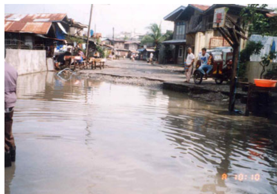
Fig. 17.34 Boundary between areas of liquefaction and no liquefaction
