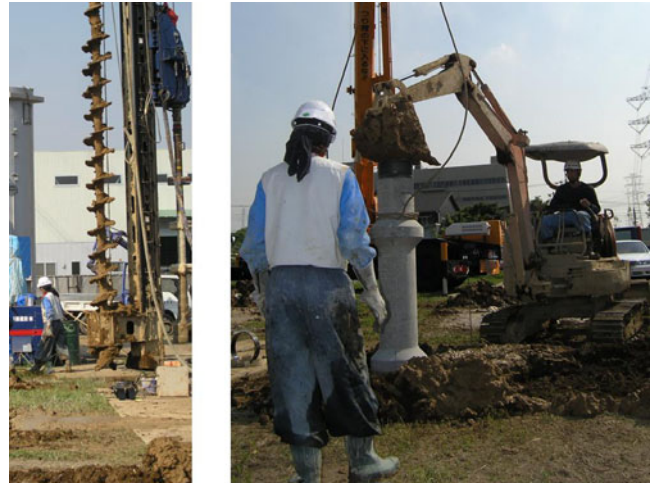
Fig. 13.32 Installation of nodular pile
