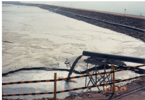
Fig. 20.23 Discharging finer tailing materials into reservoir (Lomeral in Chile)
