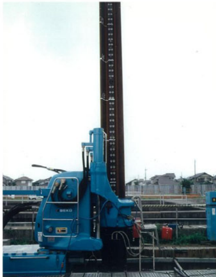
Fig. 26.91 Installation of sheet pile wall with drain (Sumitomo Metal Industries)
