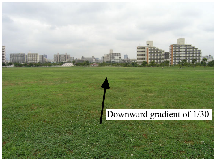
Fig. 7.13 Gentle slope of super river dike in Tokyo
