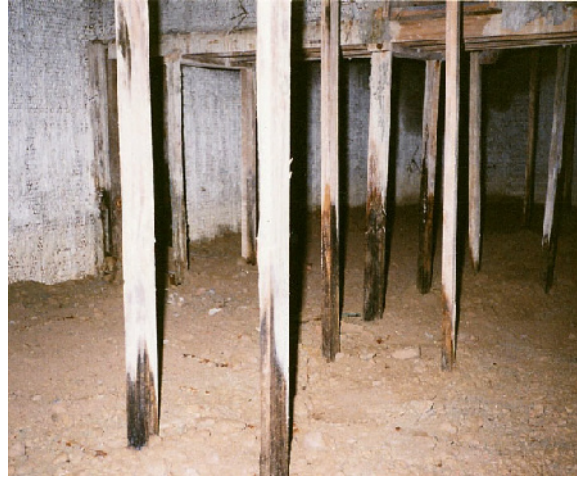
Fig. 26.113 Ground surface without sand boiling after Kobe earthquake inside lattice wall (timber columns are temporary supports during excavation (photograph by Takenaka Corporation))
