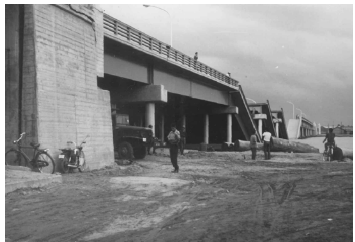
Fig. 24.64 Fallen Showa Bridge crossing Shinano River (Department of Civil Engineering, University of Tokyo)
