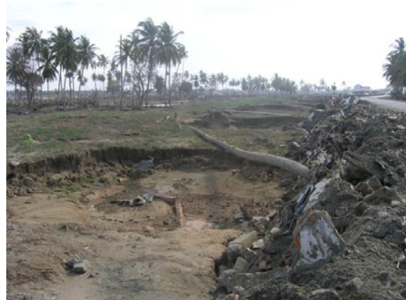
Fig. 16.61 Scoured ground behind road embankment (Banda Aceh, Indonesia)
