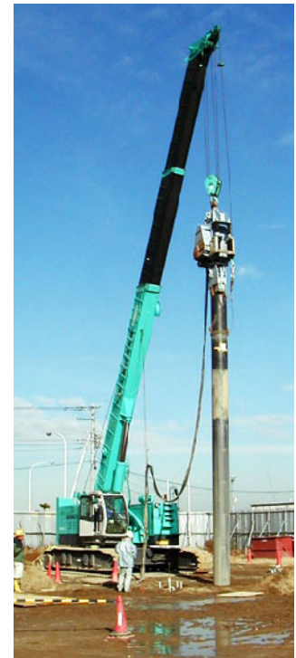
Fig. 26.98 Artificial vibration by pile driver (Zenitaka Corp.)
