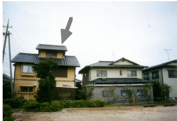
Fig. 17.59 Minor tilting of private house due to subsoil liquefaction (in Yonago City, 2000 Tottoriken Seibu earthquake)
