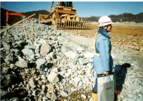
Fig. 10.51 Construction of rock fill dam
