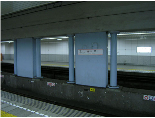
Fig. 13.6 Reinforced central columns in Kasuga Station of Tokyo Metropolitan Subway
