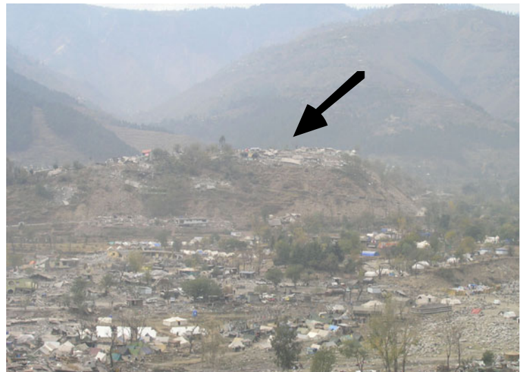
Fig. 6.33 Completely destroyed houses on terrace hill in Balakot of Pakistan during 2005 earthquake
