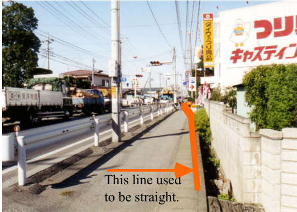
Fig. 25.20 Distortion of trench in Kasukabe which is still visible today
