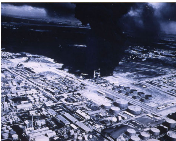
Fig. 17.69 Fire in oil refinery in Niigata (Photograph by Mr. F. Yuminamochi, JGS, 1999)
