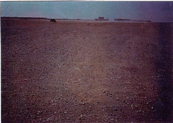
Fig. 26.71 Satisfactory effects of sand densification by dynamic consolidation in Lu-kang, Taiwan (Kaiyo Kogyo Company)
