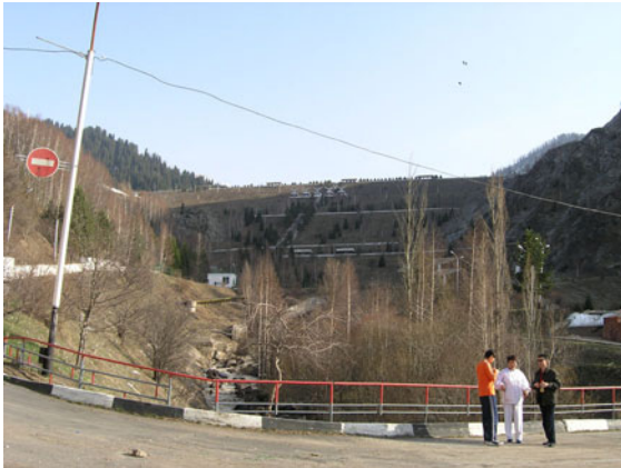
Fig. 26.6 Debris dam near Medeo of Almaty in Kazakhstan (150 m high and 530 m long)
