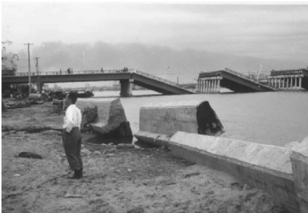
Fig. 17.1 Distortion of quay wall along Shinano River and falling of Showa Bridge in Niigata, 1964 (Department of Civil Engineering, University of Tokyo)
