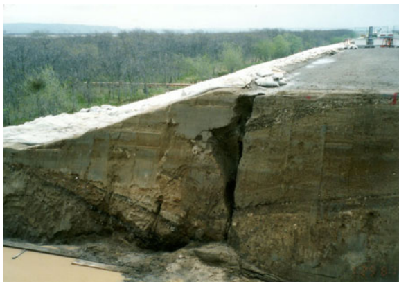
Fig. 17.10 Excavation of damaged Tokachi-river dike
