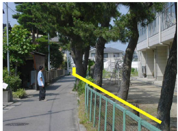
Fig. 25.30 Dislocation of pine trees due to lateral ground displacement in Ohgata, Niigata
