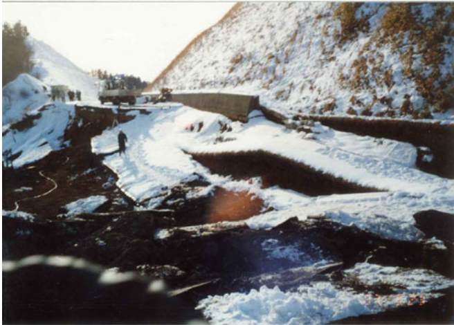
Fig. 14.43 Failed shape of Itoizawa road embankment in 1993
