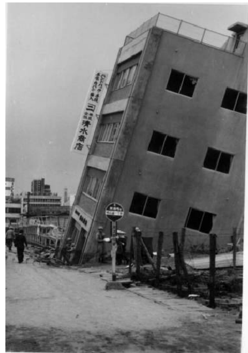
Fig. 17.2 Subsidence and tilting of building in Niigata (Department of Civil Engineering, University of Tokyo)
