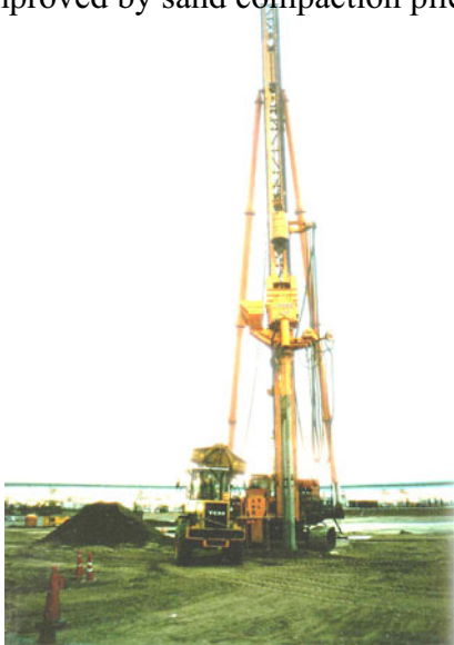
Fig. 26.52 Machine for construction of sand compaction pile
