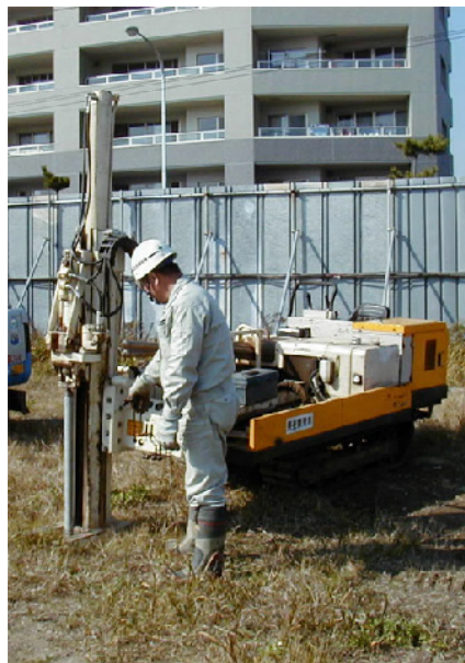
Fig. 26.97 Installation of screen pipe (Zenitaka Corporation)
