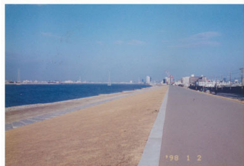
Fig. 26.107 Reconstructed shape of Yodo River dike in Osaka
