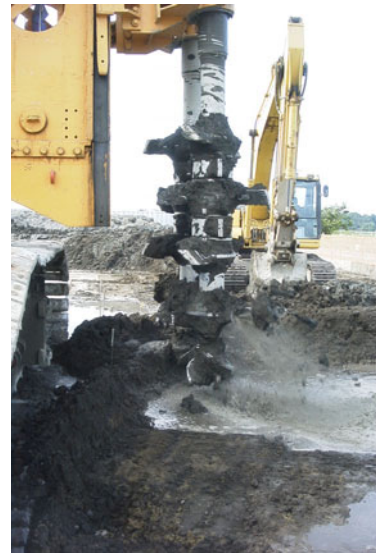
Fig. 26.105 Mixing tip of deep mixing machine under water flushing for cleaning
