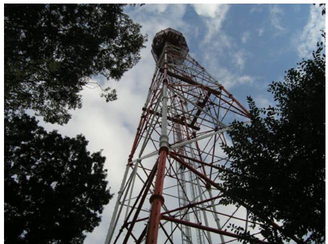
Fig. 23.18 Data transmission tower in Kodaira, Tokyo
