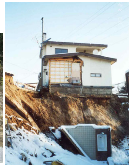
Fig. 14.10 Slip failure of fill part in cut-and-fill area (Midoriga-oka in Kushiro)
