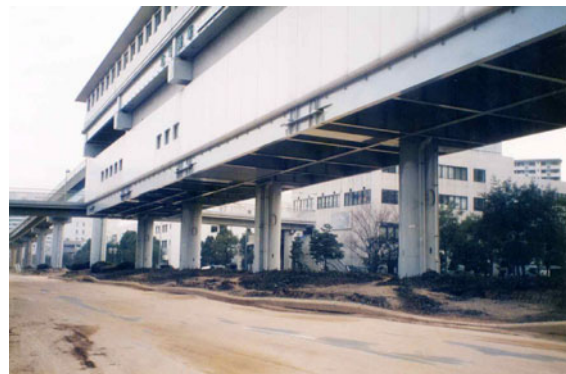
Fig. 17.31 Ground subsidence after liquefaction in Port Island, Kobe, 1995
