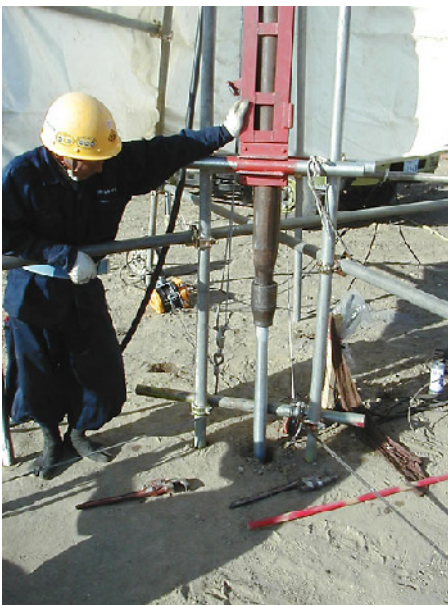
Fig. 26.97 Installation of screen pipe (Zenitaka Corporation)
