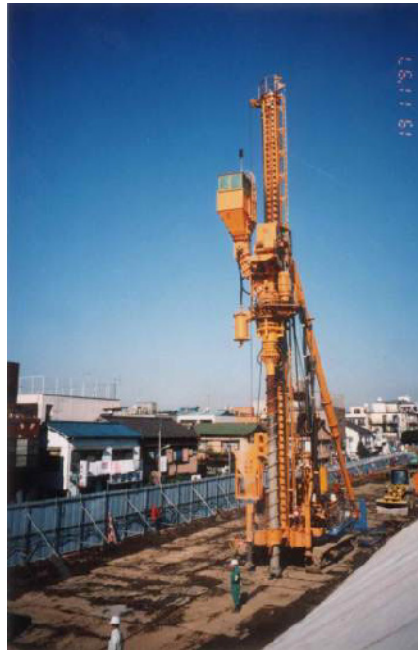
Fig. 26.86 Construction machine for gravel drain
