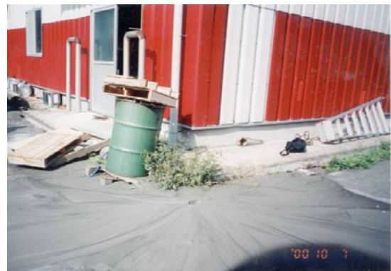
Fig. 17.39 Boiled sand in Takenouchi Industrial Park
