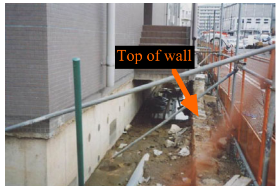
Fig. 24.83 Building foundation which was protected by underground walls from effects of lateral soil flow (Shimagami Pumping Station, Kobe; Photograph by Prof. Koseki)
