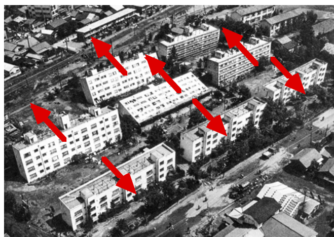
Fig. 17.6 Inclined apartment buildings in Niigata (Niigata Nippo Newspaper, 1964); arrows added by the author show direction of tilting
