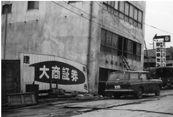
Fig. 17.50 Subsidence of building in liquefied area in Niigata, 1964 (Department of Civil Engineering, University of Tokyo)
