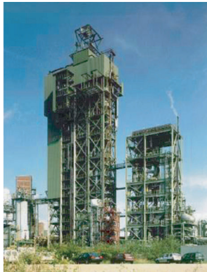
Fig. 8.1. HTW plant in Berrenrath, Germany
