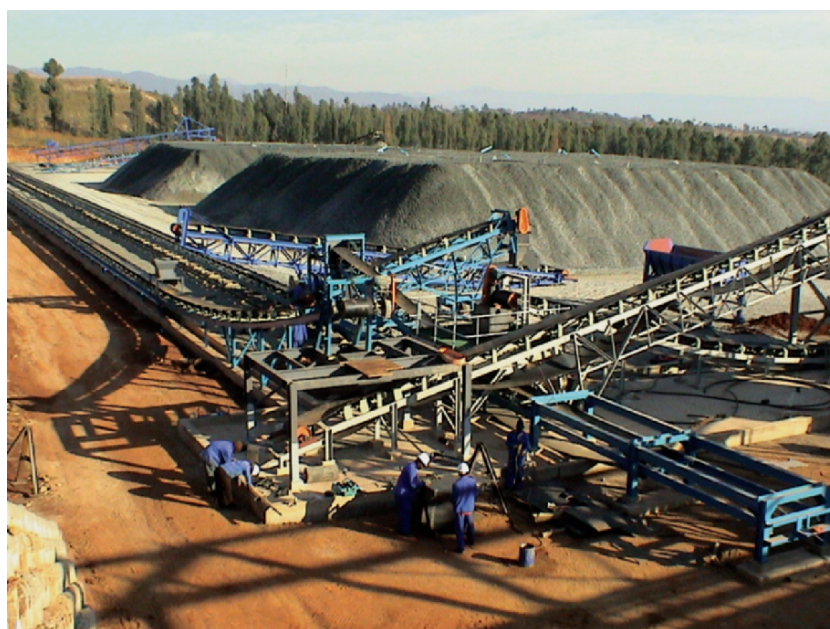
Fig. 5.6. General view of the Agnes GEOCOAT® plant
