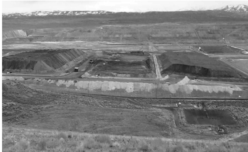
Fig. 6.1. Newmont whole-ore heap-biooxidation facility
