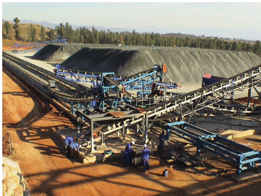
Fig. 5.6. General view of the Agnes GEOCOAT® plant
