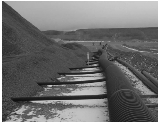
Fig. 6.5. Aeration laterals and header
