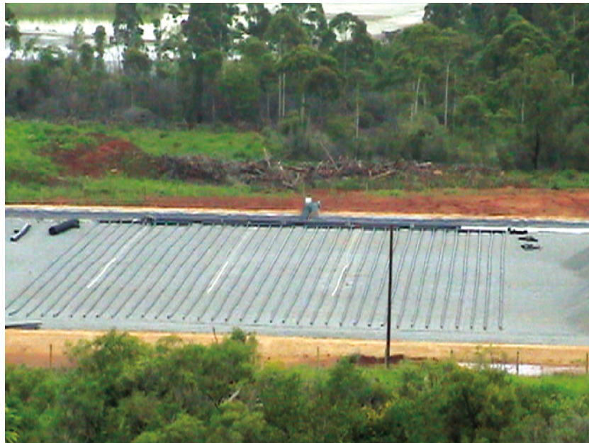
Fig. 5.5. Air supply fan and distribution system. Note the pad liner
