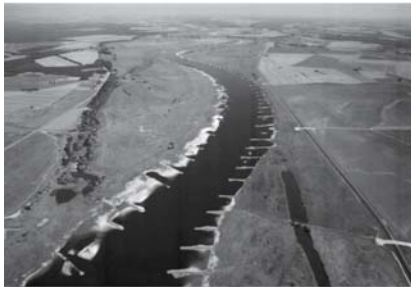
River Elbe with groyne fields
