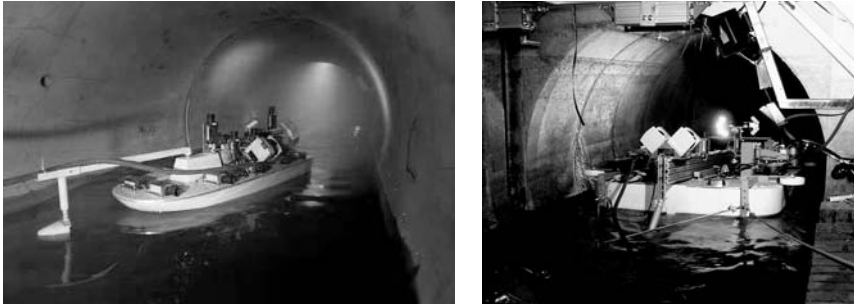
Fig. 1. Spy prototype and test of the swimming inspection system in a real sewer
