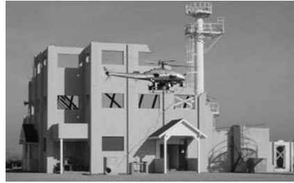
Fig. 2. The DART Collapsed Structure Rescue Training Site located in Mountain View, CA.
