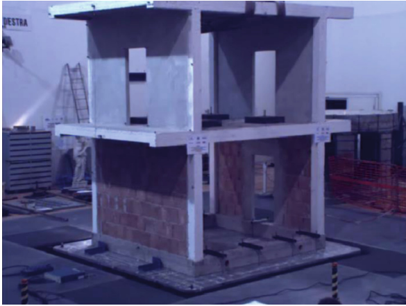
Fig. 4. The reinforced concrete structure (from the original Video 2 [9]).
