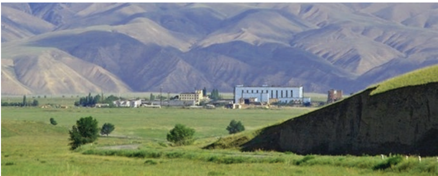
Fig. 13.3 A general view of the “Makmalzoloto” Plant
