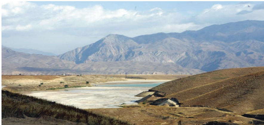
Fig. 13.4 Tailing pond in “Makmalzoloto”
