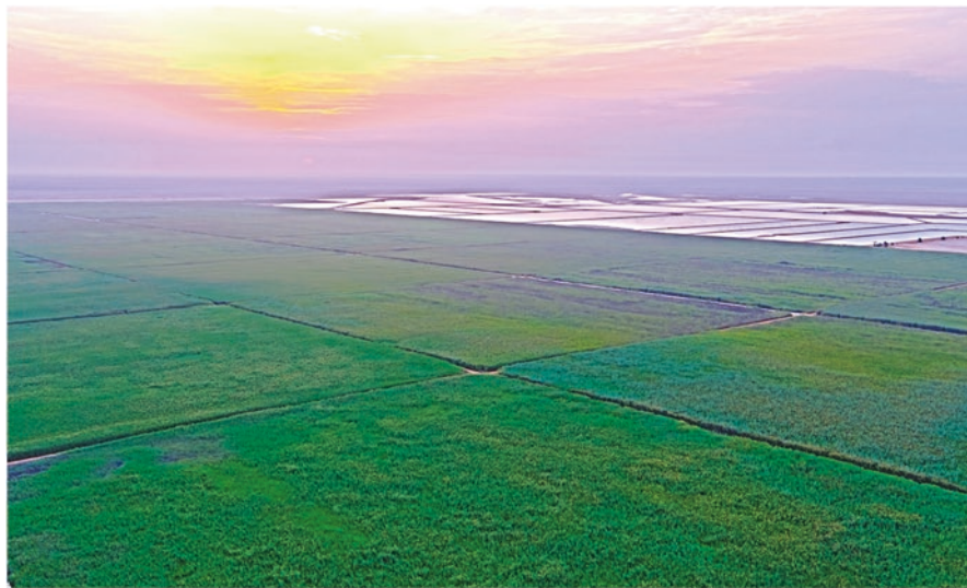
Fig. 6.6 Aerial view of the produced water treatment plant (i.e., constructed wetland cells and evaporation ponds) in the desert of Oman (photo: courtesy of BAUER Resources)
