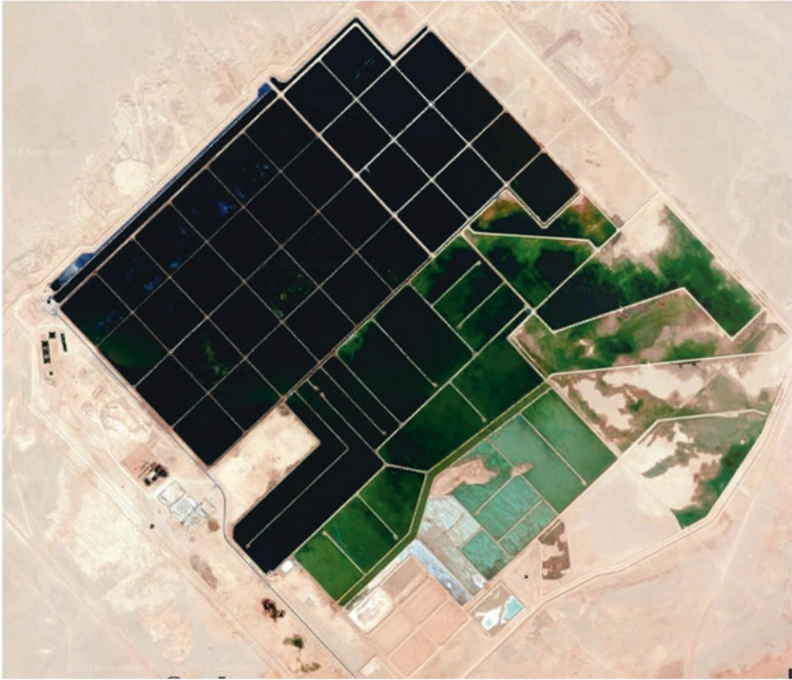
Fig. 6.4 Satellite view of the produced water treatment plant in Oman (photo: Google Earth; image accessed: May 13, 2018)
