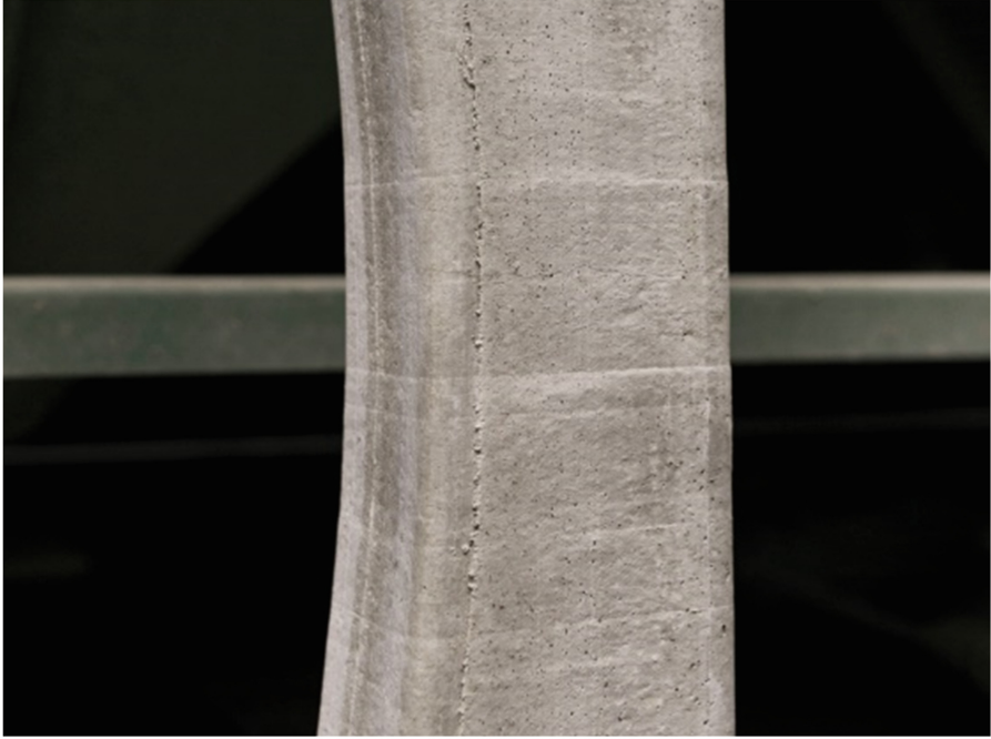
Fig. 2. Result of column produced with wooden formwork with coated with polypropylene scales, using shaping strips of scaled polypropylene. The result of the surface shows ripples and traces from the shaping strips on the left side.
