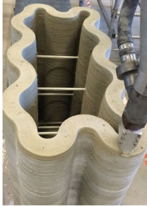
Fig. 4. Test element during printing
