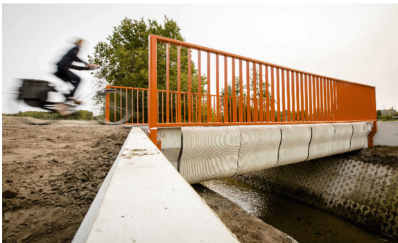
Fig. 18. Completed bridge at the opening. (photo: Kuppens fotografie)
