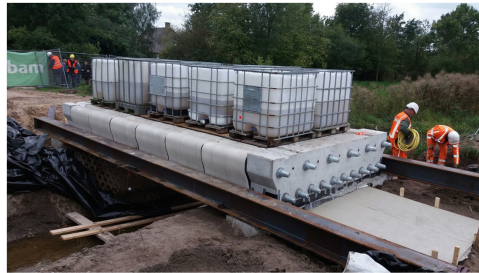
Fig. 17. In-situ testing of the bridge with water-filled containers.
