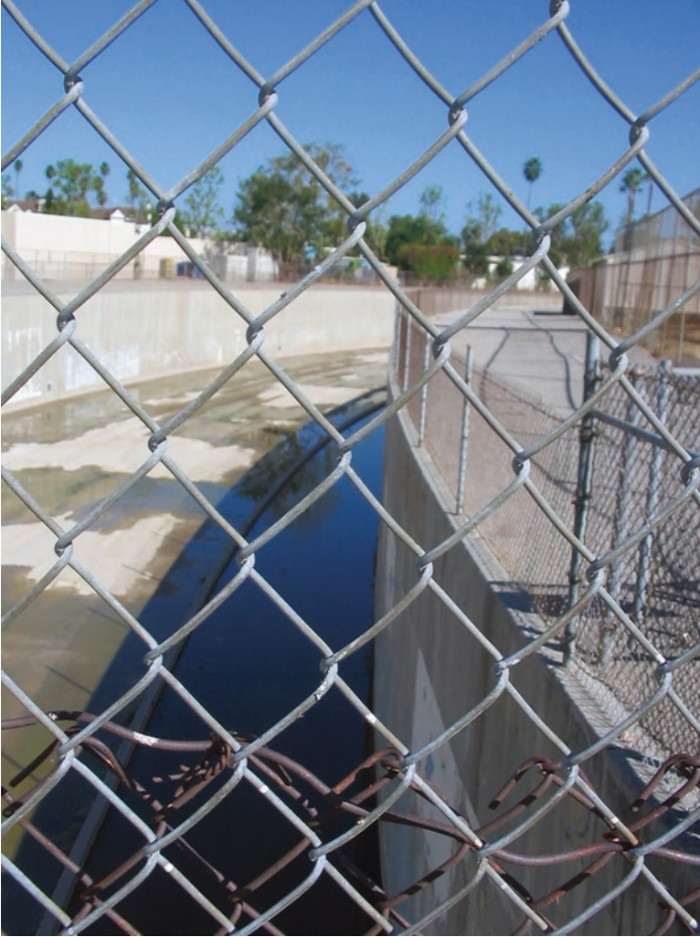
Fig. 3.8 The Forsaken River. After it was channelized in the 1950s, the Los Angeles River looked more like a “deserted freeway” than a river. Unable to access the river, many Angelenos grew up unaware that Los Angeles had a river at all. (Photograph by Irene J. Klaver)
